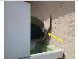
Properly sized and angled kickout flashing noted at the roof junctions throughout. This is a favorable condition. It is suggested to reseal all locations with a stucco approved sealant at this time.
