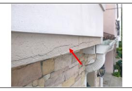
Severe cracking noted along the front right corner of the overhang. This can lead to moisture intrusion if not sealed/repaired.
