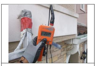
Mid moisture and firm substrate (possible framing) at the crack along the overhang at the time of inspection.
