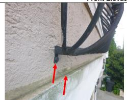
The accent bands are noted to be hard coat build outs. These are potential points of possible moisture intrusion if not maintained. It is suggested to seal the top and sides of all bands, as well as the railing attachments.
