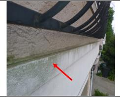
Surface staining noted throughout the front elevation. This is a common condition with stucco. It is suggested to use a light power wash with a solvent-based solution to help remedy this condition. It is recommended to repaint the home with an elastomeric paint every 8-10 years.
