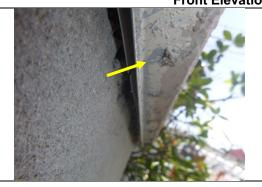
The base of the stucco walls terminates with a weep screed and proper clearance above grade. This is a favorable condition.
