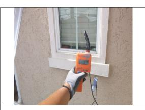
Low-to-mid moisture and firm substrate (possible framing) below the front elevation windows at the time of inspection. This is favorable.
