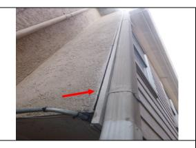
A separation crack noted along the stucco and siding transition. This can lead to moisture intrusion and possible underline issues. It is suggested to seal along all locations noted with this deficiency.
