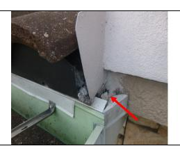
A small opening noted at the corner of the roof junction. This can lead to moisture intrusion and underline issues. It is suggested to seal all locations noted with this deficiency.
