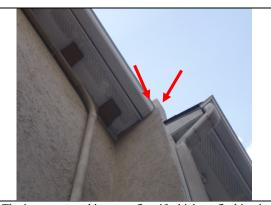
The inspector could not confirm if a kickout flashing is installed at this roof junction. It is suggested to have a stucco contractor verify the flashing at this location.
