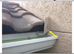
The roof junction at this highlighted location has a properly sized and angled kickout flashing (probe 1). This is favorable. It is suggested to seal all flashings at this time and every 2-3 years.
