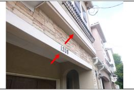
The front overhangs are closed in with stucco & have no drainage accessory. This can lead to trapped moisture and possible future damages. To help prevent future issues it is suggested to install drainage accessories at all locations noted with this deficiency.
