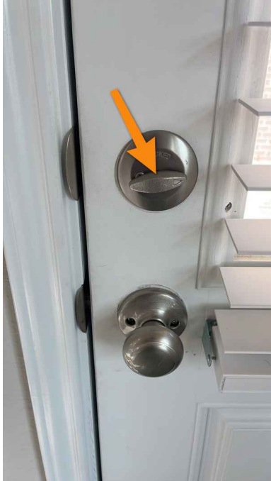
Backdoor from primary bedroom
