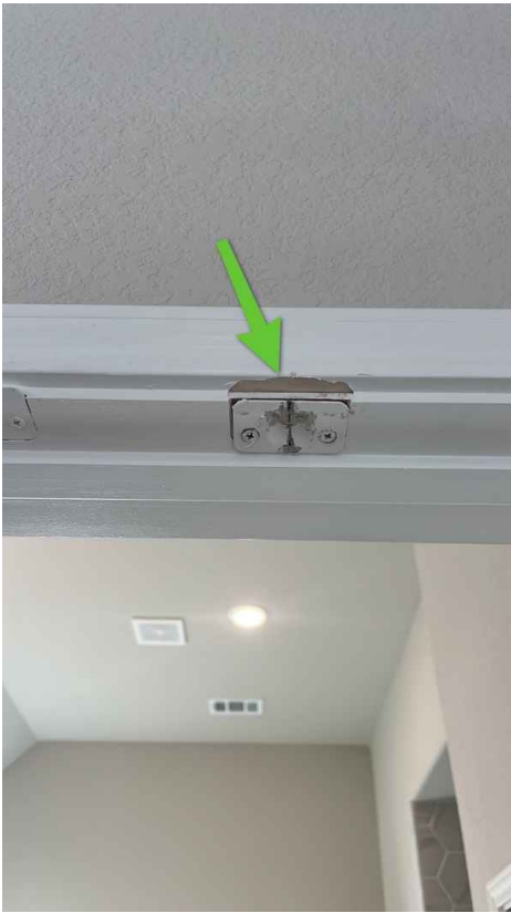
Priamry bathroom door
