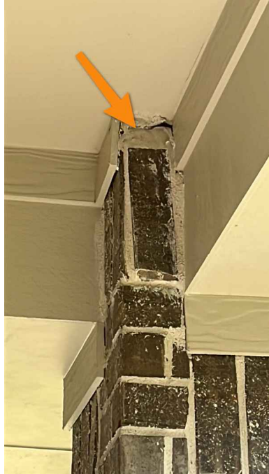
Rear- back patio area
