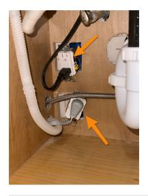
2: Non-GFCI Outlets Near Sink ASafety Hazard Kitchen Need to be changed to GFCI as it's within 6 feet of the faucet
