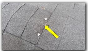
☑ Shingles lifted up and not properly laying down / sealed in some areas.
