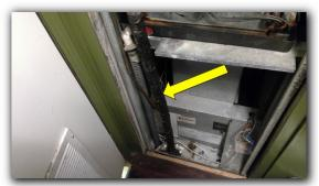
☑ Lack of GFCI operable exterior receptacle near unit for technician per current code.
