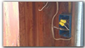
☑ Electrical wiring that has not been installed in a Usual and Customary Building Practice standard manner. Installed outside of the wall cavity. Installed on top of sheetrock.
