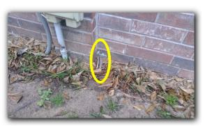
☑ Evidence of arcing or excess heat, see exterior panel box.
