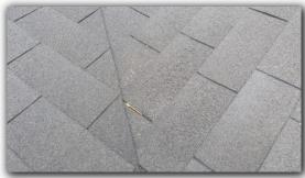
☑ Flashing is incorrectly installed. Diverter flashing needed at all roof / wall intersections.
