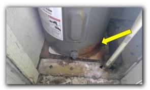
☑ Leakage / Floor rot observed around water heater and water heater appears to be in danger of collapsing through the floor.
