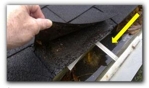
☑ Torn, damaged, perforated or missing shingles.
