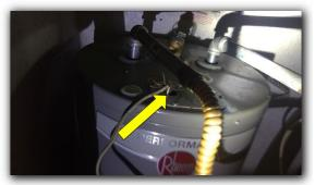
☑ Water heater electrical connection is not professionally installed per usual and customary building practices and is unsafe in current condition.
