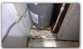
☑ Inspection of water heating equipment was limited due to inadequate access and wood rot damaged flooring.
