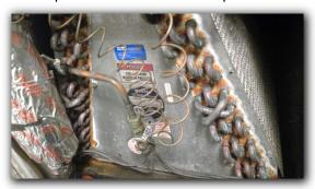
☑ Refrigerant lines not properly insulated at evaporative coil (wrong thickness per current code)
