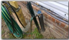
☑ Proper insulation needed on exterior exposed water lines / plumbing
