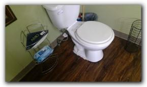
☑ Toilet plastic anchor bolt covers missing, see primary bathroom.
