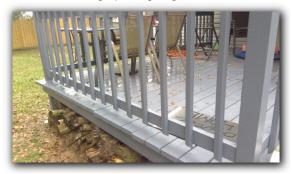
☑ Improper dimensions of exterior stair risers: riser height cannot vary more than 3/8" from the lowest riser to the top riser per current code.
