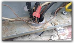
☑ Exposed wiring present in electrical panel box.
