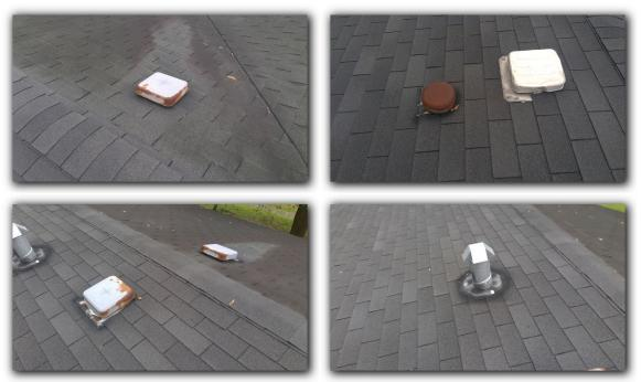
☑ Exposed nails at multiple locations need to be properly caulked / sealed.
