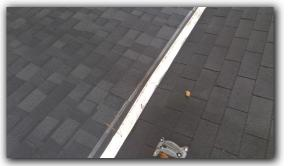
☑ Significant signs of roof deterioration were observed. Gravel coming loose, pitted surfaces, fiberglass threading showing at edge of shingles, shingle corners are turning up. Would recommend contacting a roof professional to make any further recommendations and / or repairs.
