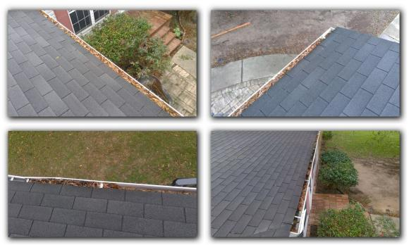
☑ Gutters / downspouts observed to be damaged / dented at one or more locations.
