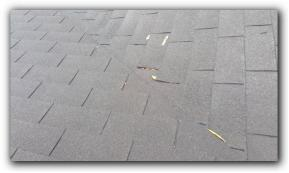
☑ Inappropriate roof covering for slope of the roof. Dimensional / tab shingles should not be used in low slope roof applications. Consult manufacturer's specifications for details, see rear porch addition.
