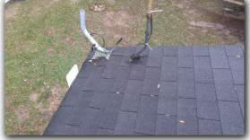
☑ Vent roof jacks missing or improper installation.
