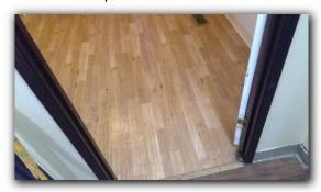
☑ Higher and lower areas observed in floor surface noticeable when walking across the floor.
