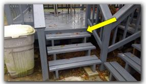
☑ Hand railing at exterior stairs not at proper height: Current code requires handrail to be installed 34" to 38" measured vertically from the bullnose of the stairs
