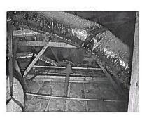
We did vent the master bath vents into the affic so there would not be one single vent pipe coming out of the roof in the front roof.
