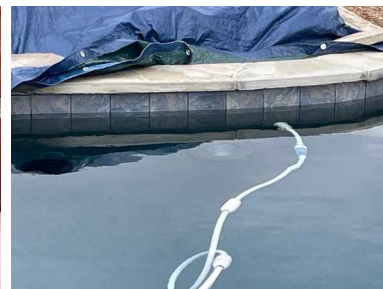
Pool light responded to GFCI
