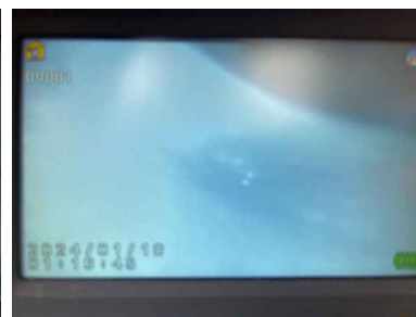
General view obstructed by water
