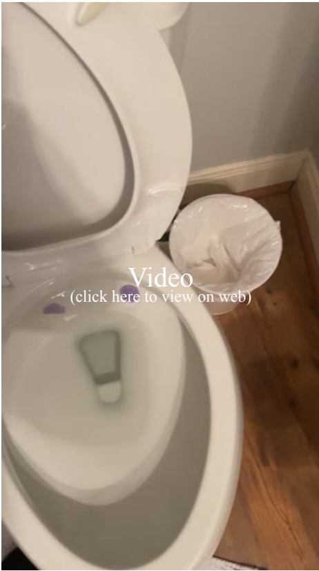
Half bathroom fixtures running
