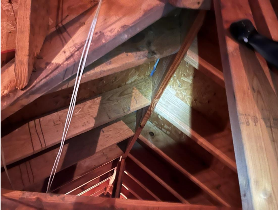
Photograph 5: Attic Framing – Good condition. No twisting, pulling or cracked structural members.
