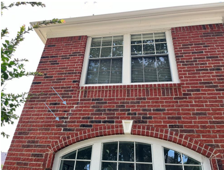
Photograph 2: Repaired cracks in front brick veneer.
