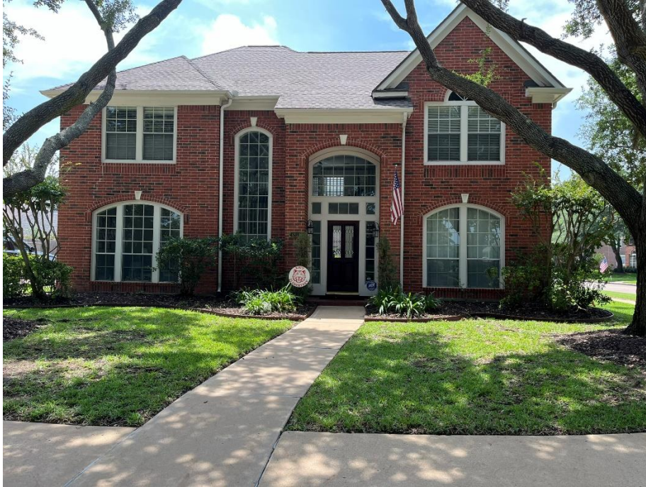
Photograph 1: Overview of front of residence.
