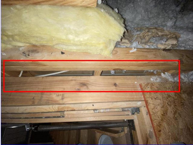
E. Item 7(Picture) Next to attic opening
