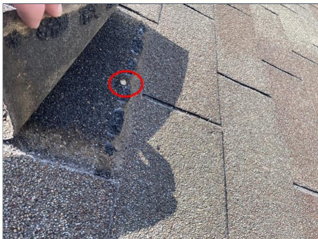
C. Item 11(Picture) Nails driven into adhesive strip
