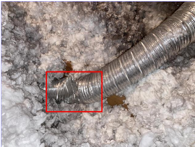
F. Item 2(Picture) Laundry room vent
