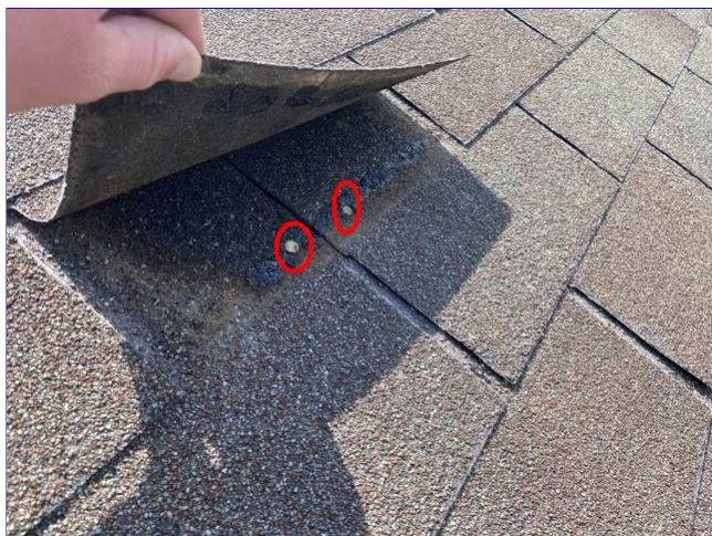
C. Item 12(Picture) Nails driven into adhesive strip
