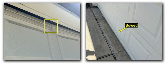
Deterioration observed at the garage door frame.
