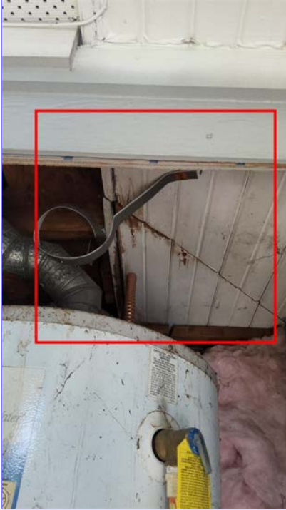
F. Item 4 (Picture) bedroom 1
