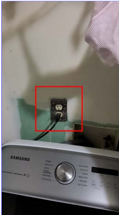
B. Item 4 (Picture) utility room
