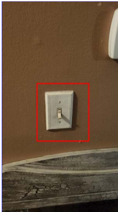
B. Item 10 (Picture) hall way
