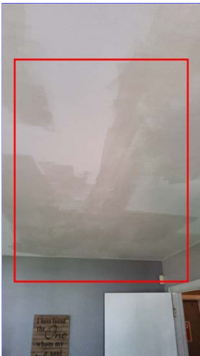
F. Item 13 (Picture) living room
