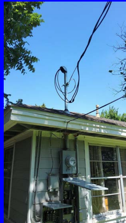
electrical meter backyard
