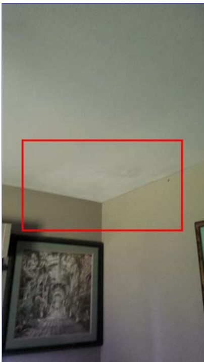
F. Item 15 (Picture) bedroom 2
