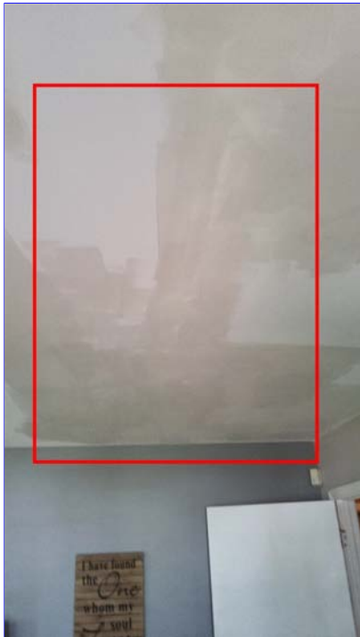
F. Item 8 (Picture) living room
