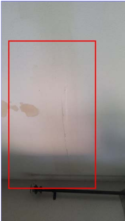
F. Item 7 (Picture) living room
