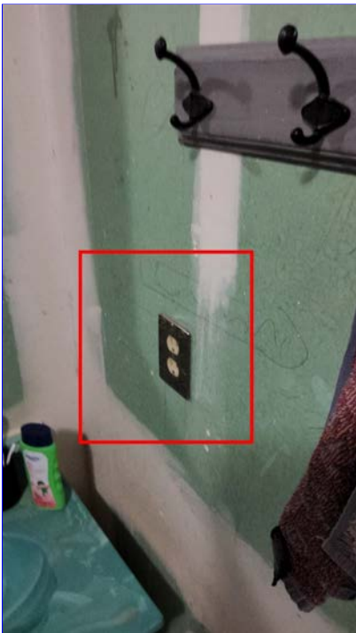
B. Item 5 (Picture) utility room
