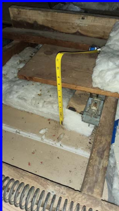
4in batt and blown in insulation
