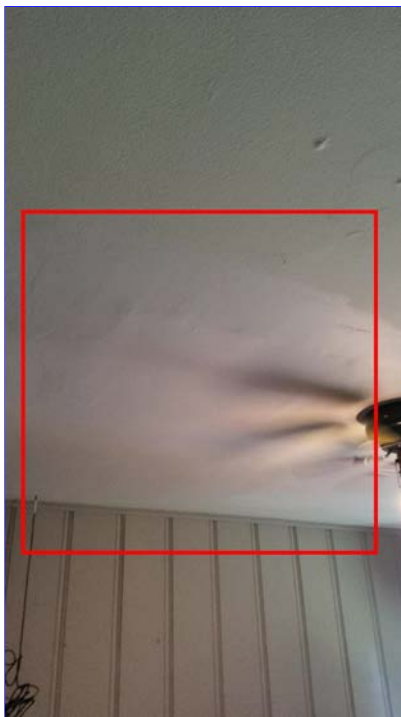
F. Item 14 (Picture) bedroom 1
