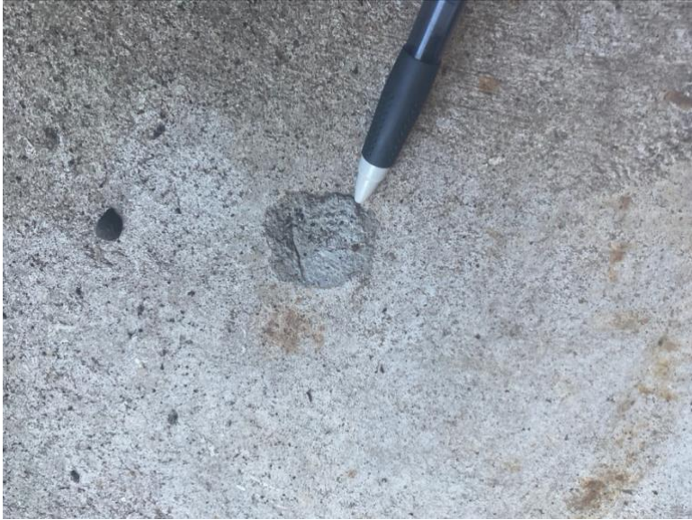
Drill Holes observed around the structure.
