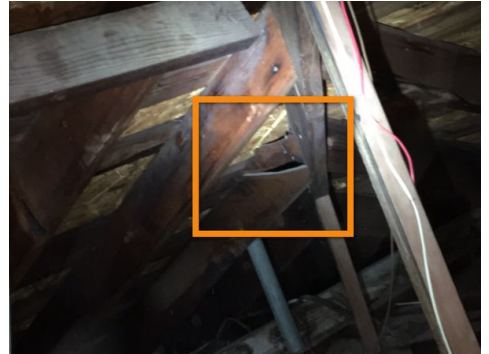
Rear of the garage
