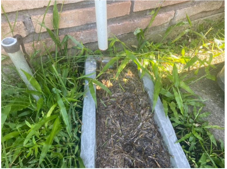
Moisture was observed due to the A/C primary drain line. Condition needs to be corrected.
