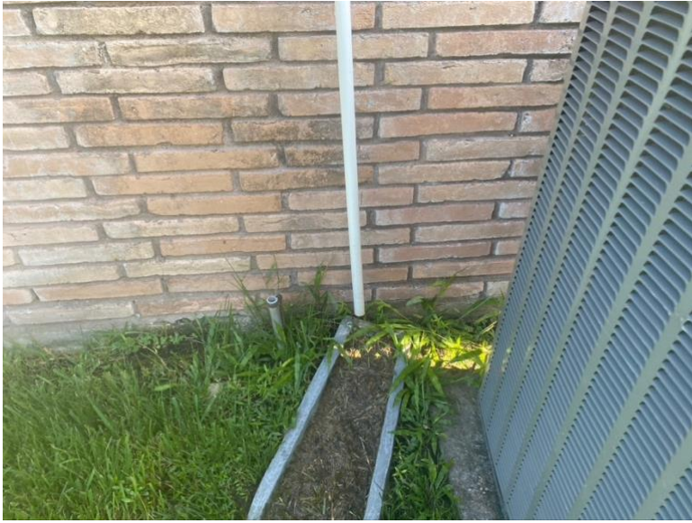
Moisture was observed due to the A/C primary drain line. Condition needs to be corrected.
