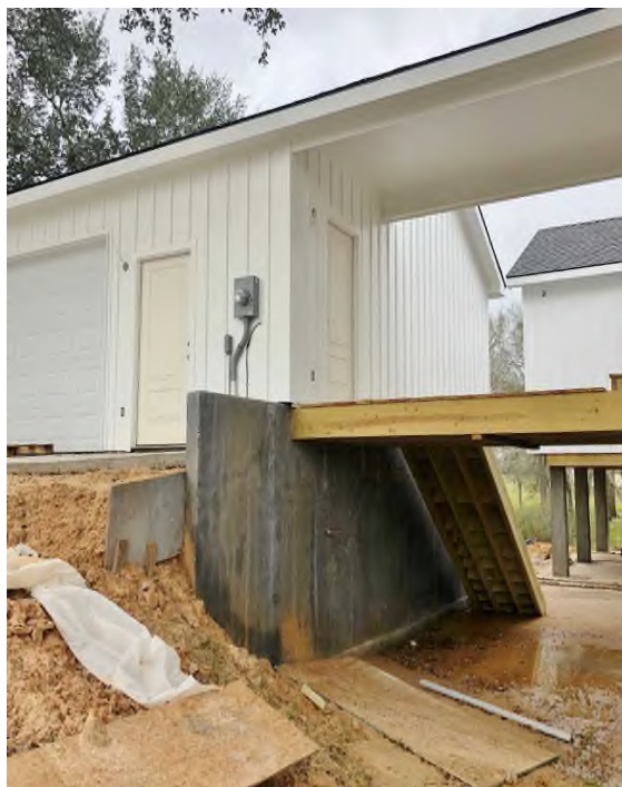
View of South side of house showing garage. (02-07-2019)
