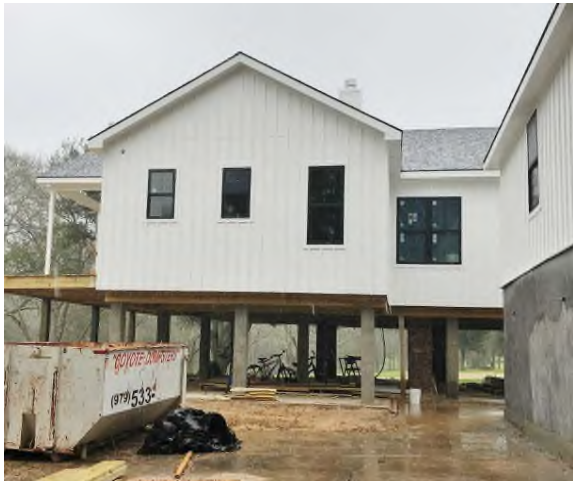
View of West side of house & North side of garage. (02-07-2019)
