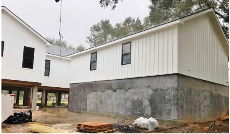
View of West side of house, showing rear of garage. (02-07-2019)
