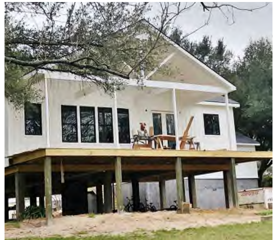
View of North side of house. (02-07-2019)
