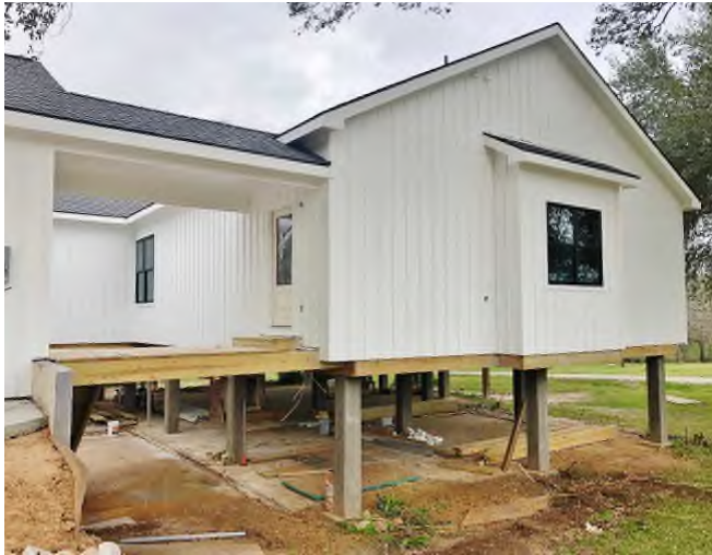
View of south side of house. (02-07-2019)
