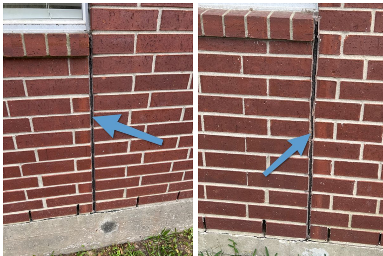
Expansion Joint - Right Side Exterior
