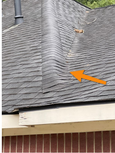
Shingles should not be woven in valleys
