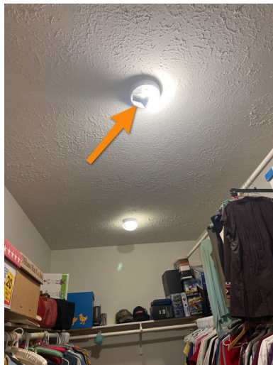
Master Bathroom Closet
