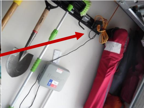
Extension cord used as permanent power
