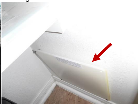
No access to pump under tub
