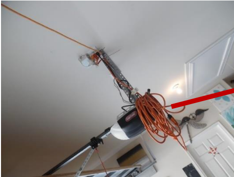
Extension cord used as permanent power
