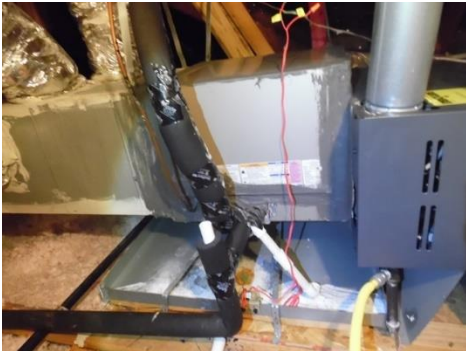
Evaporator coil
