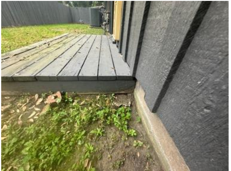
Wood to ground contact – Deck is conducive be design - Area should be monitored for insect activity
