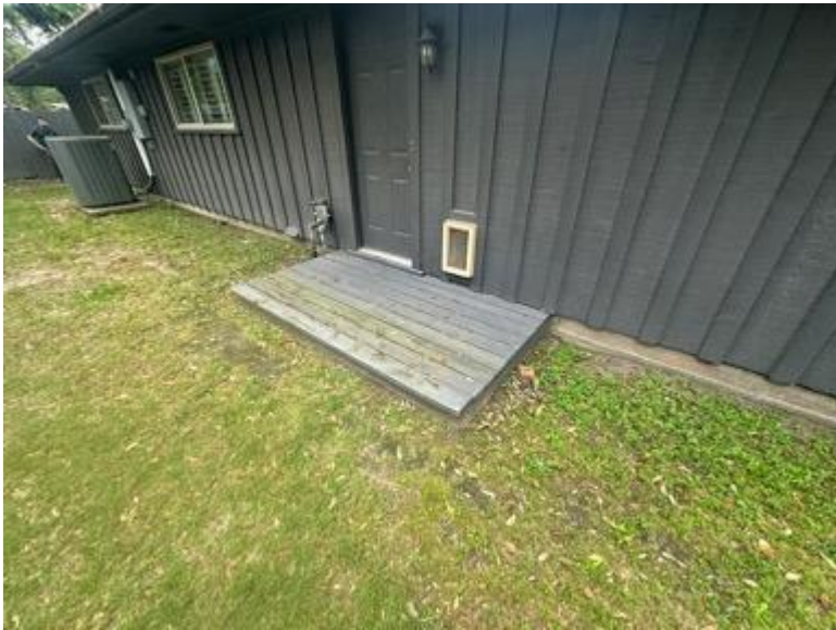
Wood to ground contact – Deck is conducive be design - Area should be monitored for insect activity
