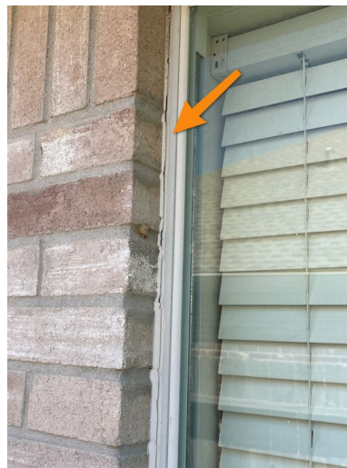
Left (window frames)
