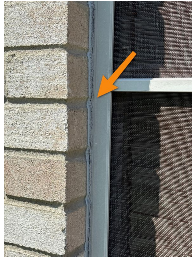
Right (Window frames)
