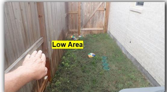
*Underground yard and/ or pool deck drainage system not tested for flow, adequacy and placement.. Did not verify yard drains operate properly and that there are no collapsed or clogged areas. Inspector (or anyone else) is unable to induce sufficient quantity of water to determine if system will operate properly when needed. Recommend observing performance during heavy rains and ensure system is maintained / cleaned.*
