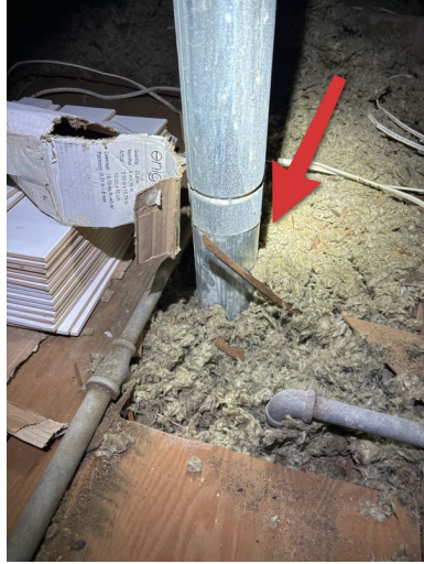
Insulation around vent
