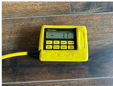
Living room (slope measurement)
