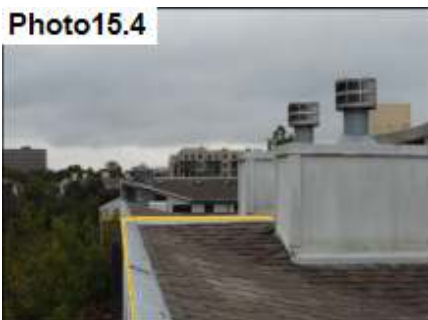
Metal Cap Termination / Seal
