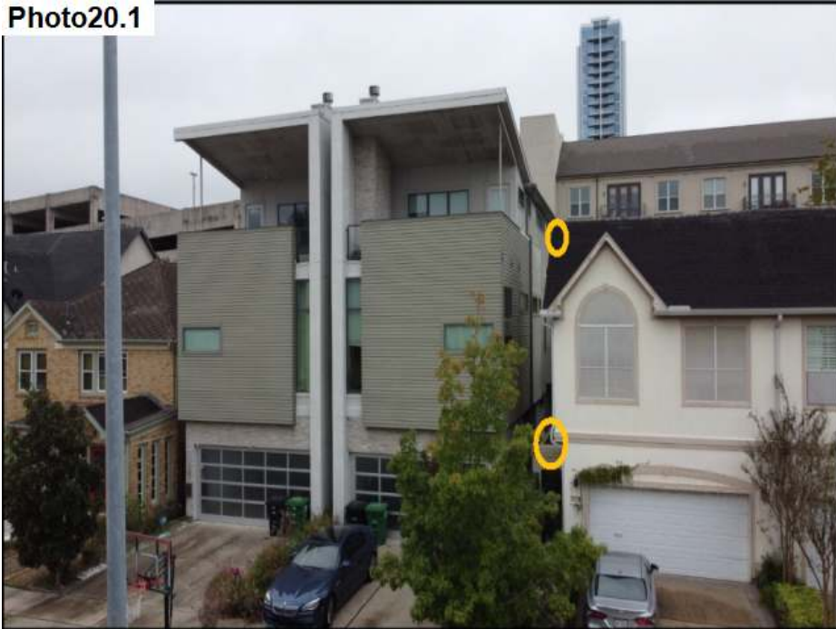
Rust stains have been removed. A new AC pan was installed.
