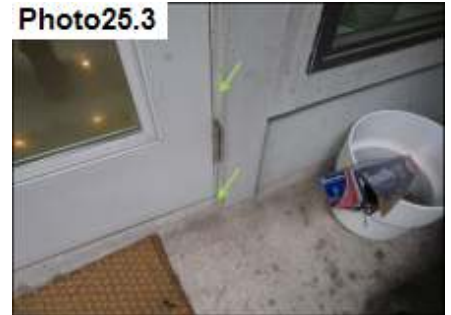
Door Trim and Miter Sealant / Seal
