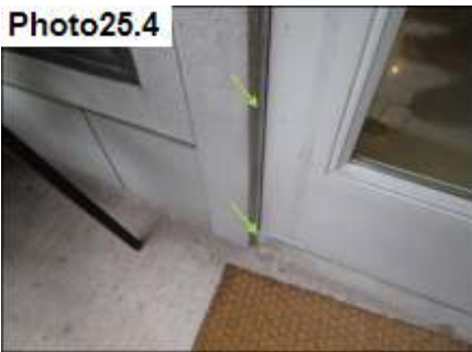
Door Trim and Miter Sealant / Seal
