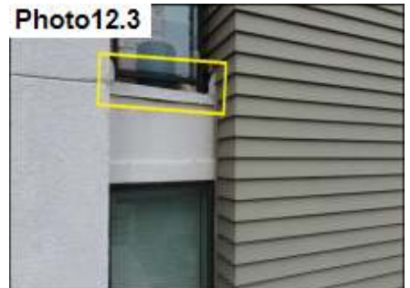
Balcony Flashing / Seal
