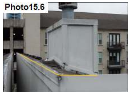
Metal Cap Termination / Seal
