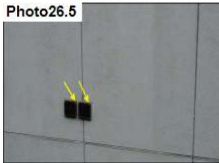
Penetration Sealants / Seal
