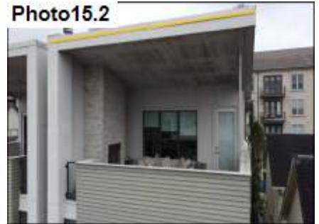
Metal Cap Termination / Seal
