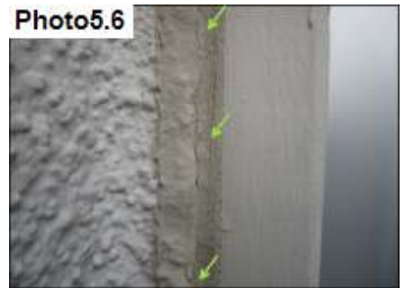
Garage Door Trim Sealant / Seal
