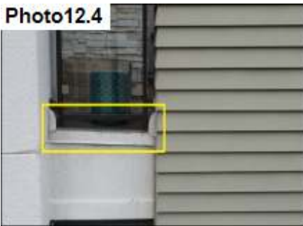
Balcony Flashing / Seal
