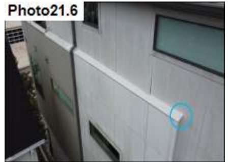
Roof Diverter Flashing and Metal Cap / Seal
