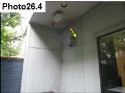
Penetration Sealants / Seal
