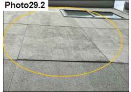
Cementitious Fiber Panel / Re-Fasten
