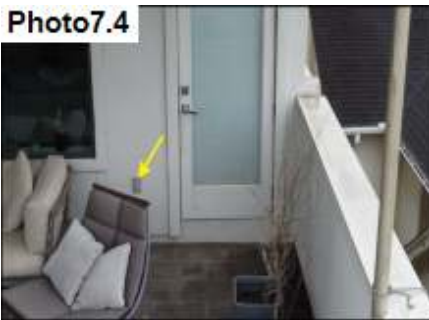
Penetration Sealants / Seal
