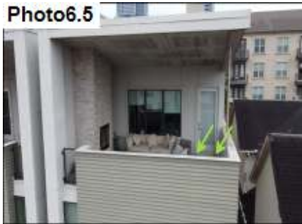
Door Trim and Miter Sealant / Seal
