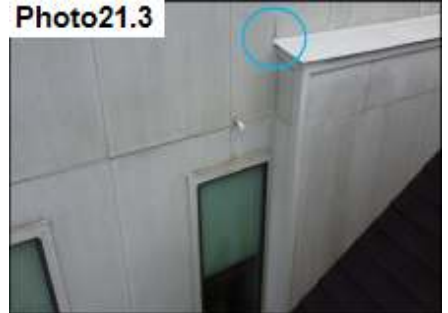
Roof Diverter Flashing and Metal Cap / Seal
