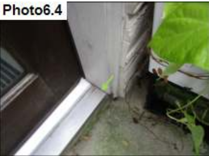
Door Trim and Miter Sealant / Seal
