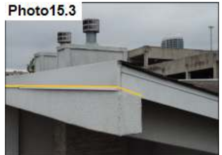
Metal Cap Termination / Seal
