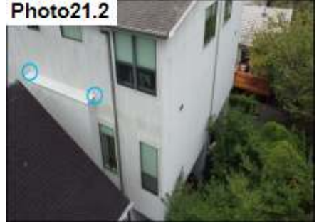
Roof Diverter Flashing and Metal Cap / Seal
