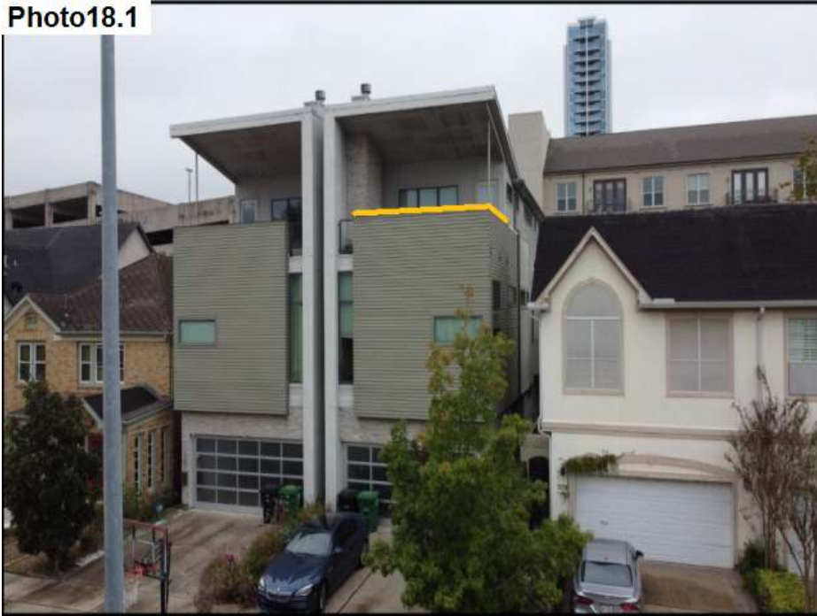
Metal cap has been sealed.
