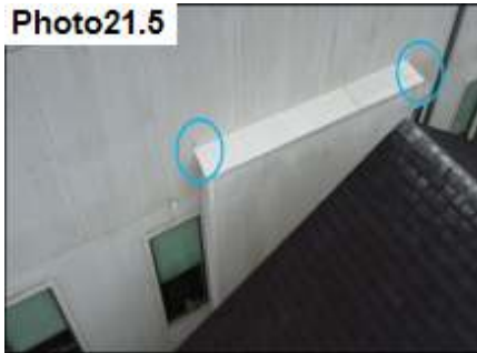
Roof Diverter Flashing and Metal Cap / Seal
