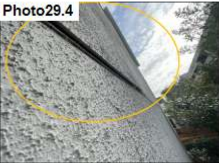
Cementitious Fiber Panel / Re-Fasten
