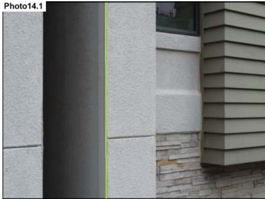
Siding & Stucco Termination / Seal
