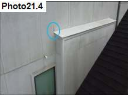
Roof Diverter Flashing and Metal Cap / Seal
