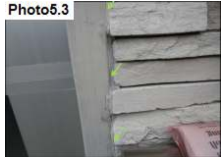
Garage Door Trim Sealant / Seal
