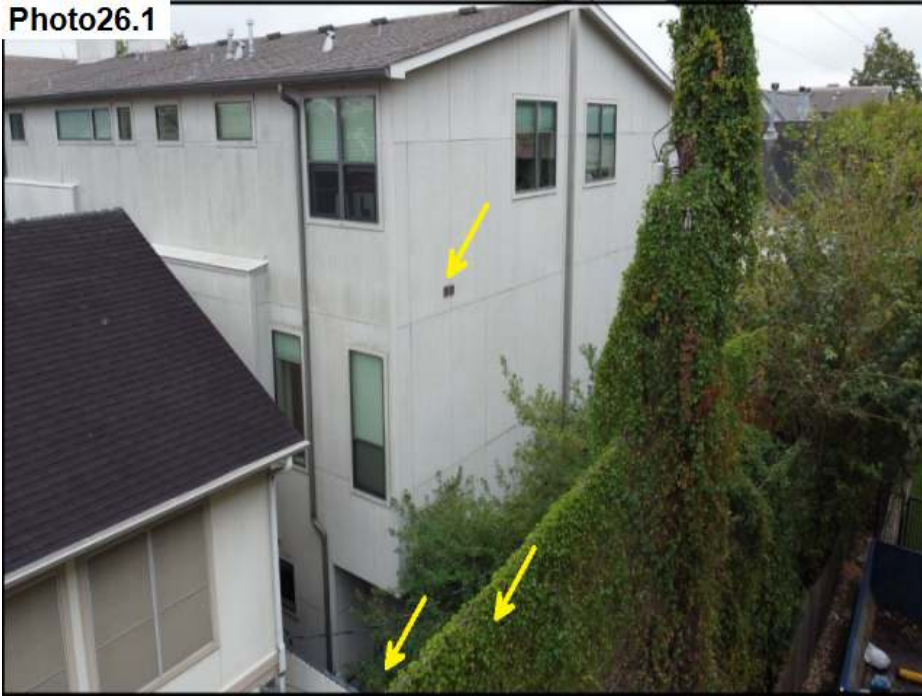
Penetrations have been sealed.
