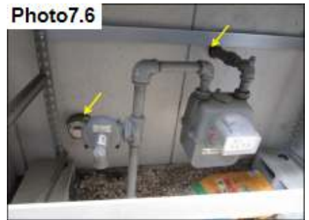
Penetration Sealants / Seal
