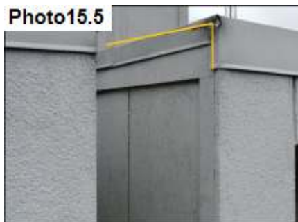
Metal Cap Termination / Seal
