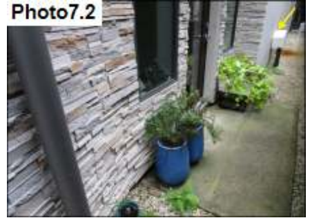
Penetration Sealants / Seal
