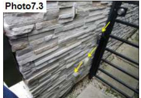
Penetration Sealants / Seal
