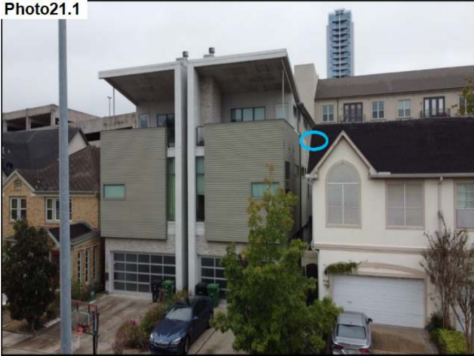
Roof diverter flashing and metal cap has been sealed.
