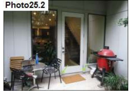
Door Trim and Miter Sealant / Seal
