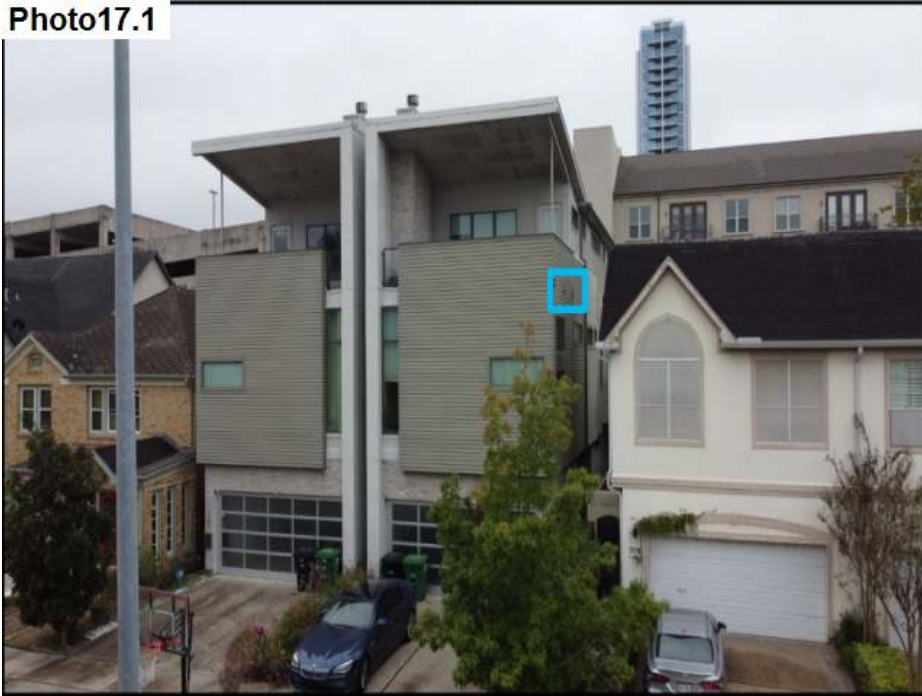
Scuppers have been sealed.
