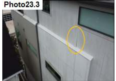
Cementitious Fiber Panel / Re-Fasten
