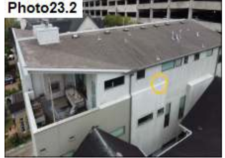
Cementitious Fiber Panel / Re-Fasten
