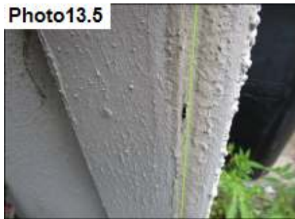
Siding & Stucco Termination / Seal
