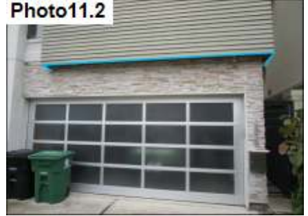
Obstructed Relief / Clean Out
