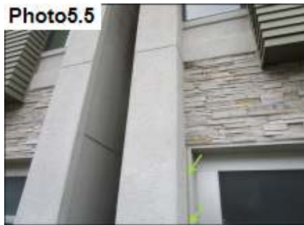
Garage Door Trim Sealant / Seal
