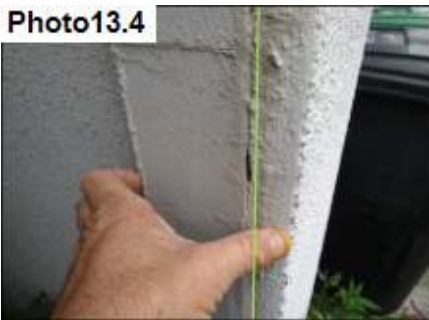
Siding & Stucco Termination / Seal
