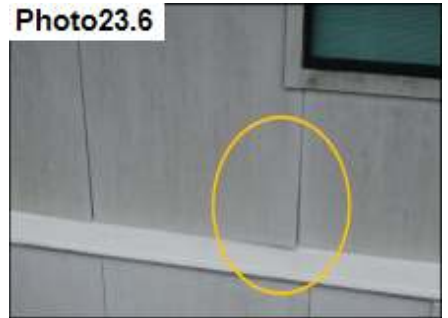
Cementitious Fiber Panel / Re-Fasten
