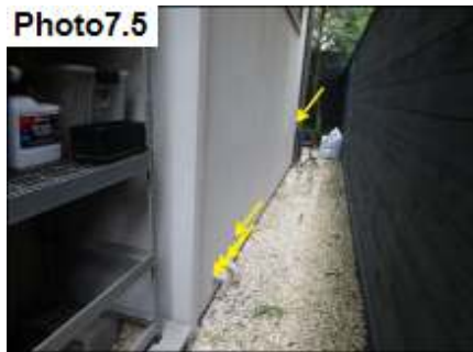
Penetration Sealants / Seal
