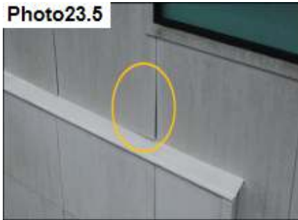
Cementitious Fiber Panel / Re-Fasten
