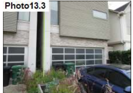
Siding & Stucco Termination / Seal
