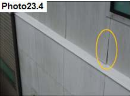
Cementitious Fiber Panel / Re-Fasten
