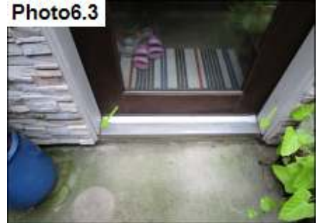
Door Trim and Miter Sealant / Seal
