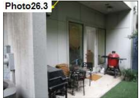
Penetration Sealants / Seal
