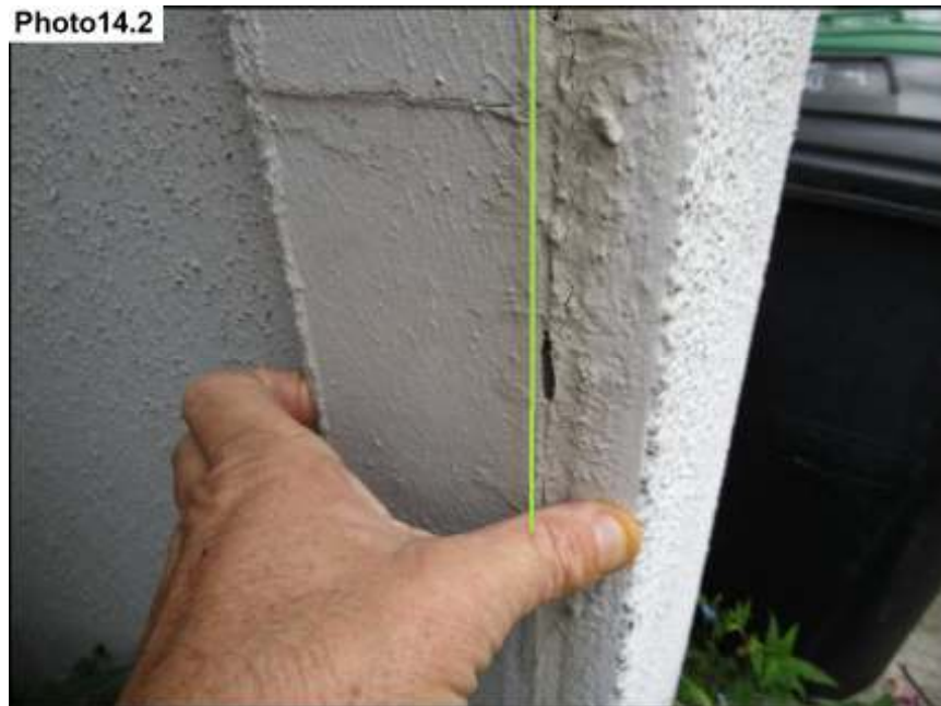
Siding & Stucco Termination / Seal
