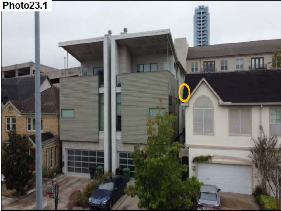
Cement panels were re-fastened/secured.
