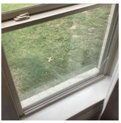
• Window does not close enough to latch, and the one window latch is loose. It is recommended to consult with a qualified contractor to evaluate and make any necessary repairs to restore proper function. (Upper Front Bedroom)
