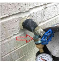
• No anti-siphon protection present on exterior hose bibs/faucets. This is a basic safety attachment to the end of faucets that will protect from a cross connection or back-sipohange into the drinking water system. (Exterior Left)
