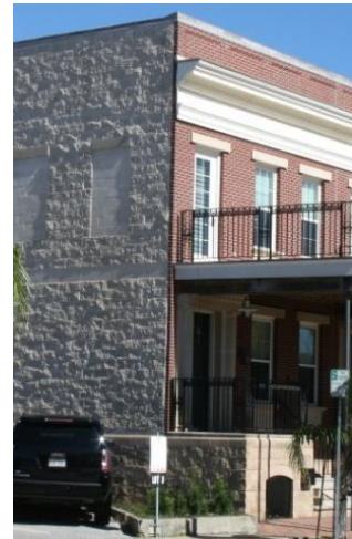
Undesirable building corner treatment
