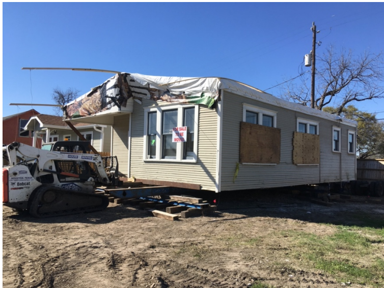
Arrival of 2/1 bungalow at 502 Dell Ct.
