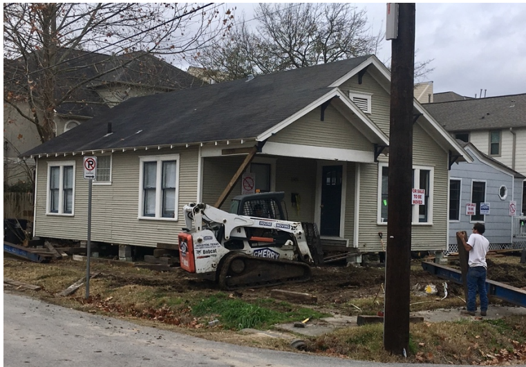
House being prepared for relocation. 1501 Malone
