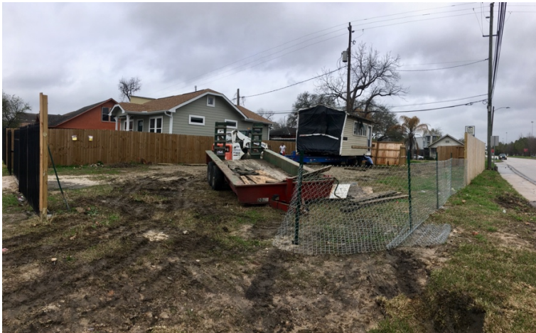
Breezeway structure was first to arrive at 502 Dell Ct location.
