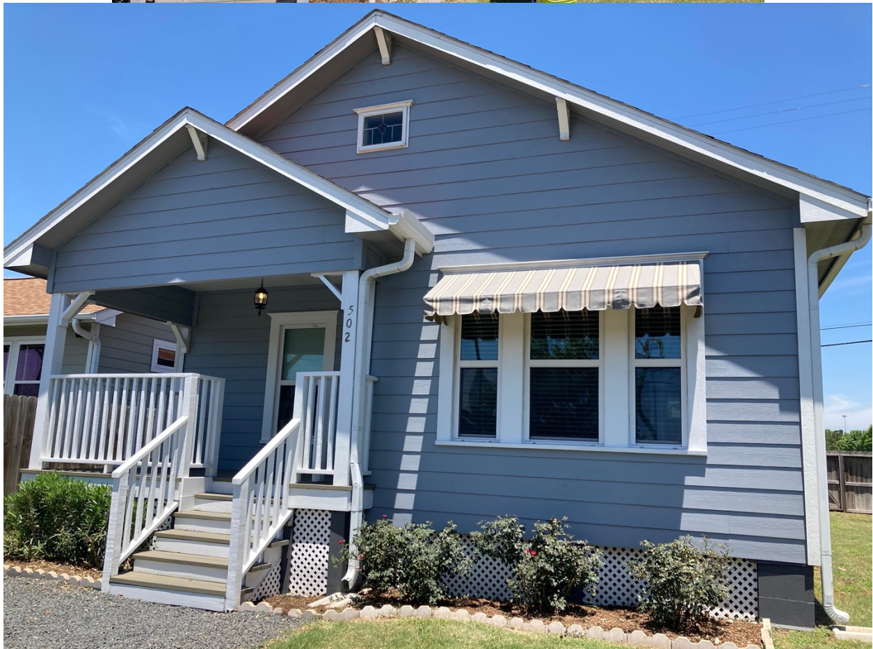
New front window awning installed May, 2024 on existing aluminum frame. Frame and awning manufactured by A.K.Hill Awning & Tent Company located in the Montrose section of Houston.
