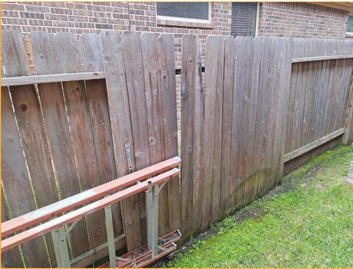
Normal wear and tear and loose pickets in areas
