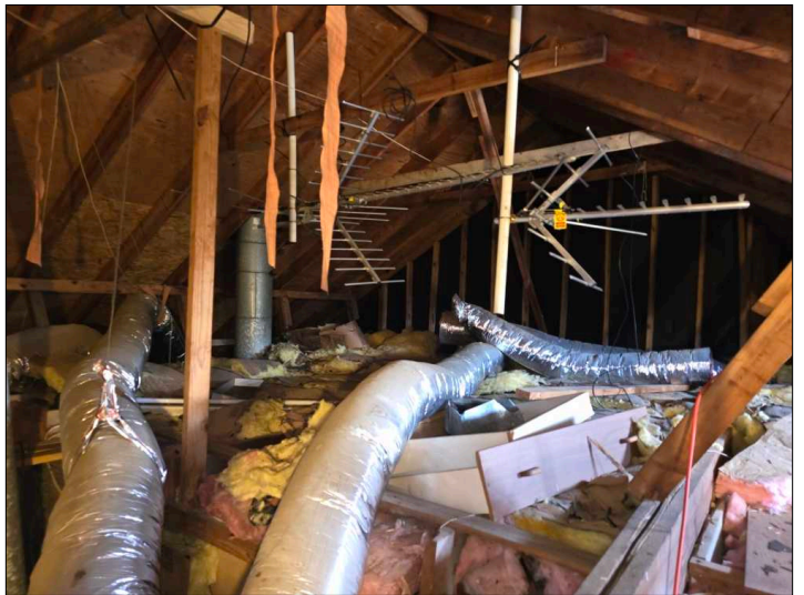
Overview of Attic.
