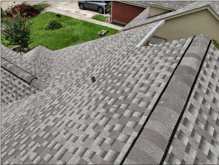
Overview of Roof.
