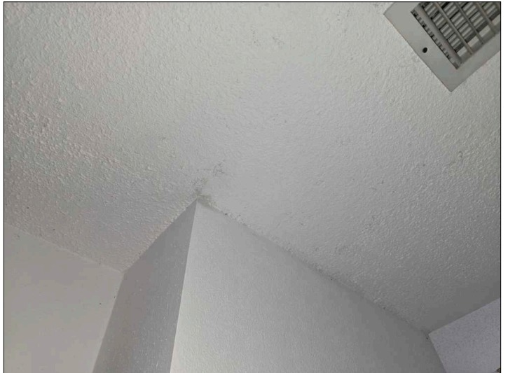
There are indications of water penetration to the ceiling evident mainly by deterioration. Unable to determine condition of the underlying materials. Mainly at - kitchen
