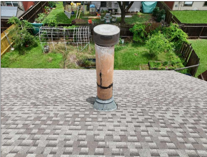
Overview of Chimney.
