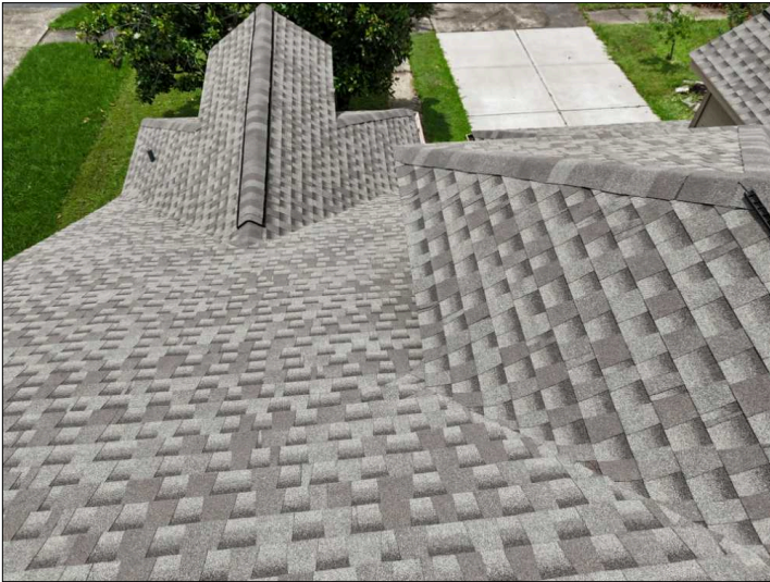
Overview of Roof.
