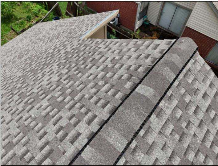
Overview of Roof.
