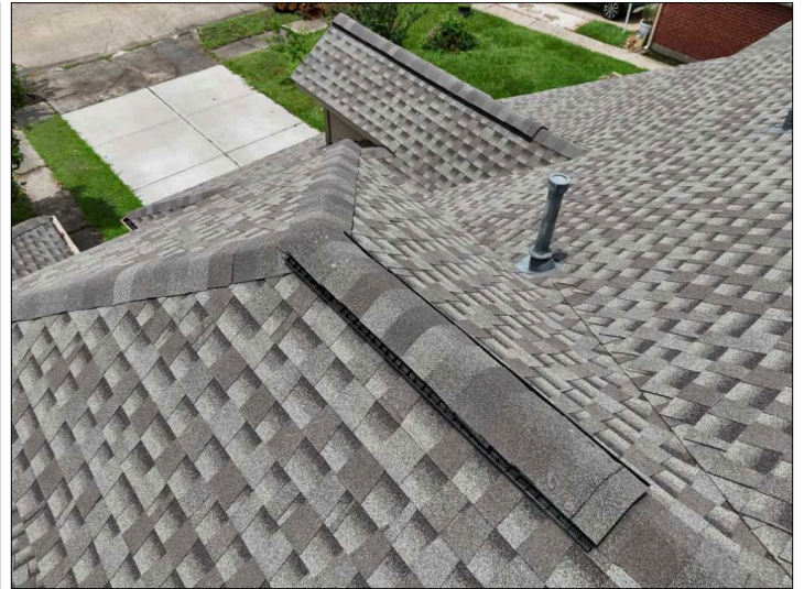
Overview of Roof.
