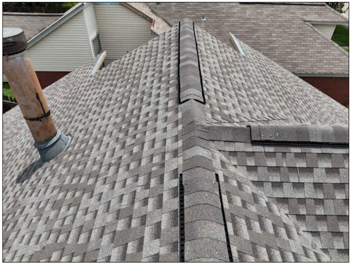
Overview of Roof.
