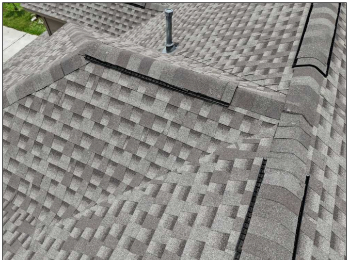
Overview of Roof.
