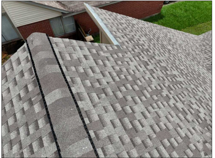
Overview of Roof.
