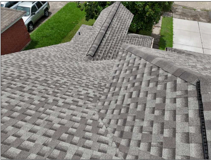
Overview of Roof.
