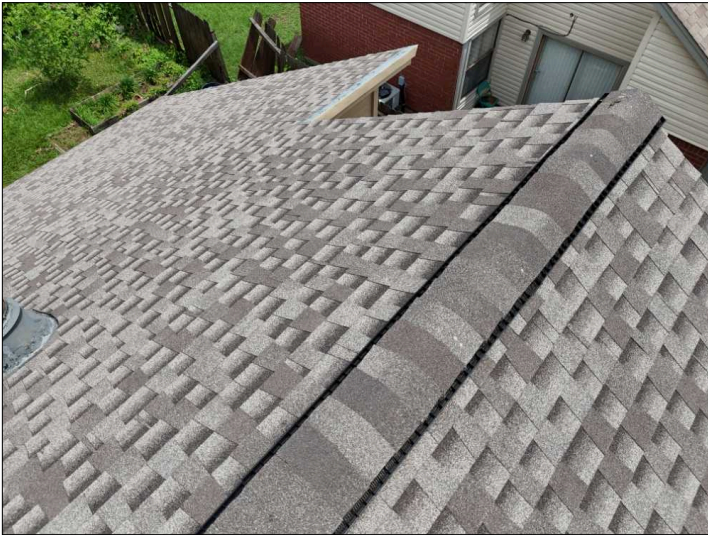
Overview of Roof.
