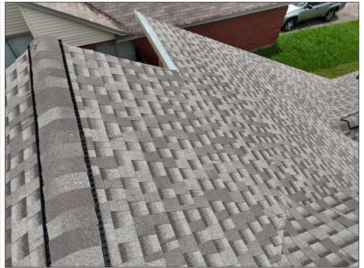
Overview of Roof.
