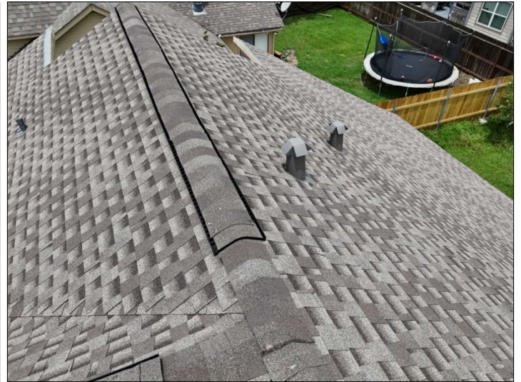
Overview of Roof.
