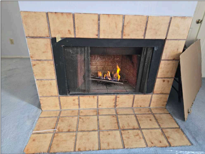
Overview of fireplace
