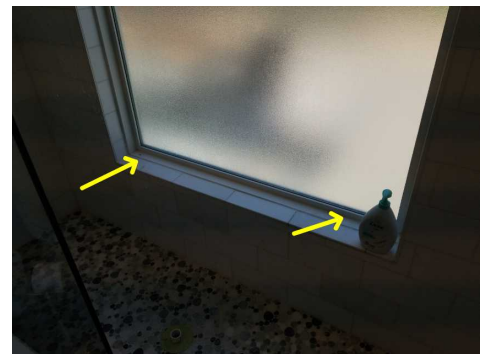
Caulk/ seal screws to prevent water damage inside wall
