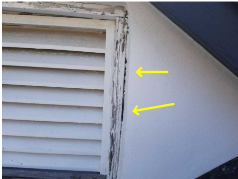
Caulk attic vent
