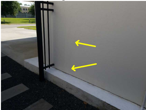
Seal cracks in stucco, West exterior
