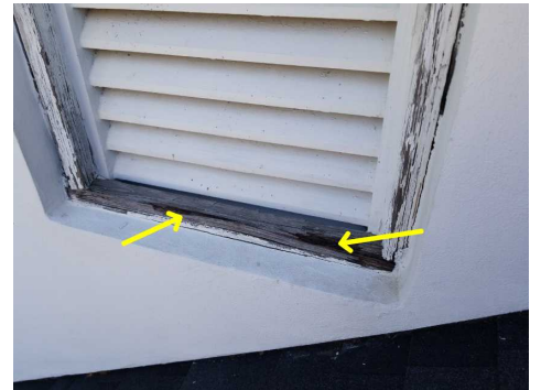
Wood rot at West attic vent
