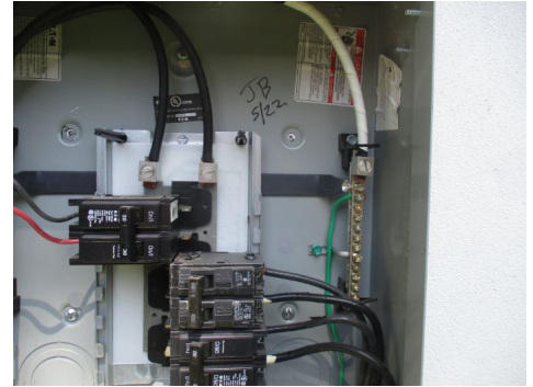
Improper wiring to sub-panel - the neutral and ground wires are not on separate bus bars as required on sub-panels.
