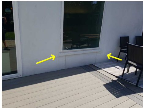
Seal stucco cracks
