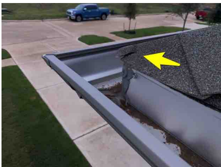
Lower roof front right corner
