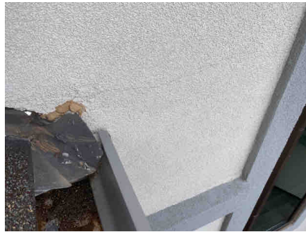
Upper wall above the garage, front left area
