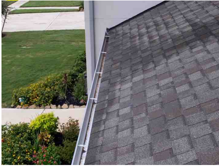
Lower roof front left
