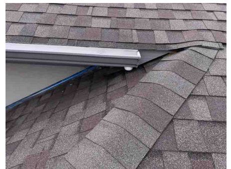
Front right upper roof
