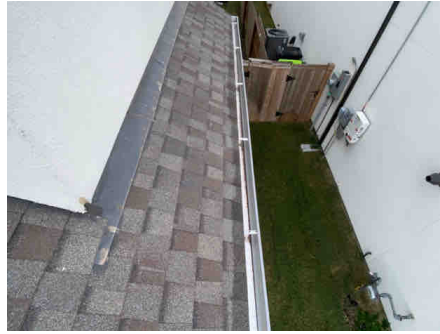
Lower roof right side
