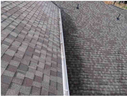
Upper roof back left at the porch
