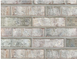
EXTERIOR BRICK + FRONT PATIO FLOOR
