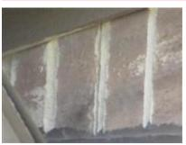
R – The front porch arch is constructed as a self supporting arch but on a flexing foundation is in need of a steel support lentil. IRC R608.8.2 Lintels
