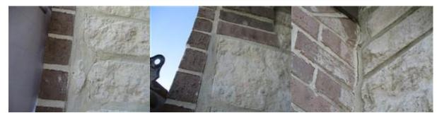
R – Seal other open expansion joints. This prevents water intrusion into the wall cavity.
