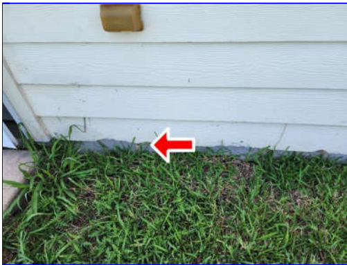
E. Item 18(Picture) Rear
