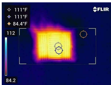
Area #1 Temperature at Register
