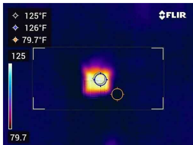
Area #1 Temperature at Register
