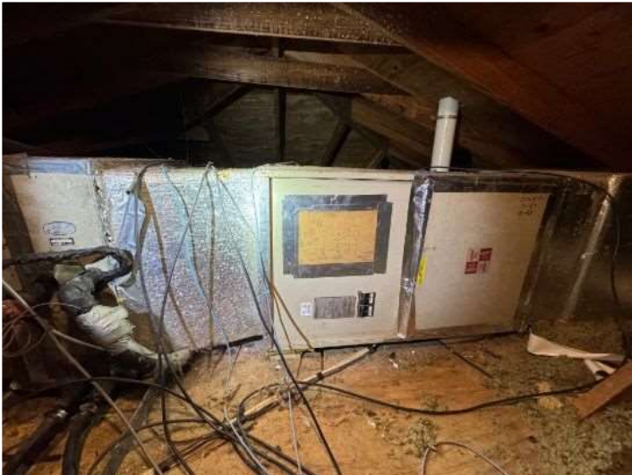
Furnace installed as per standards
