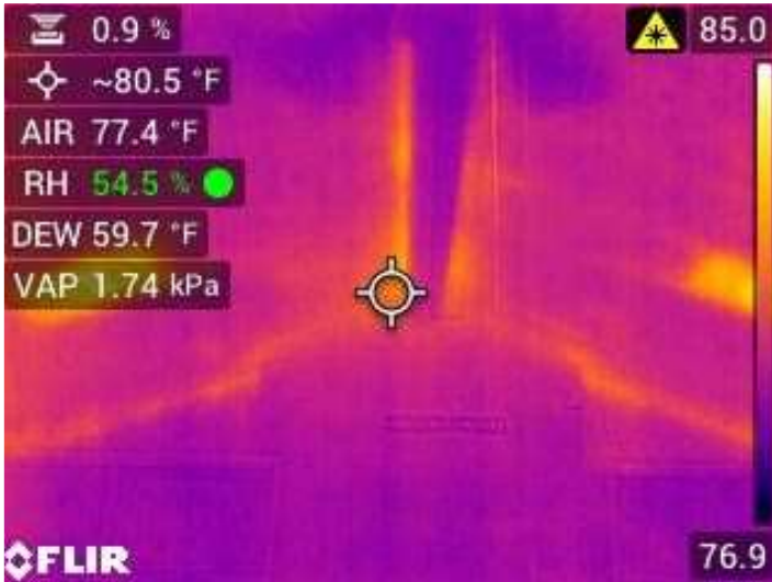
Thermal scanning - Living area
