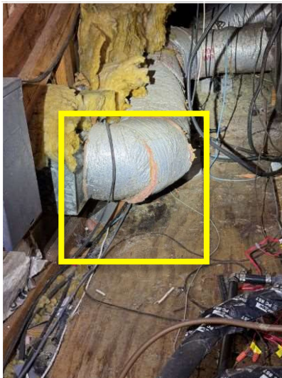
Condensation on HVAC ducts in attic - Active moisture from attic to living area ceiling
