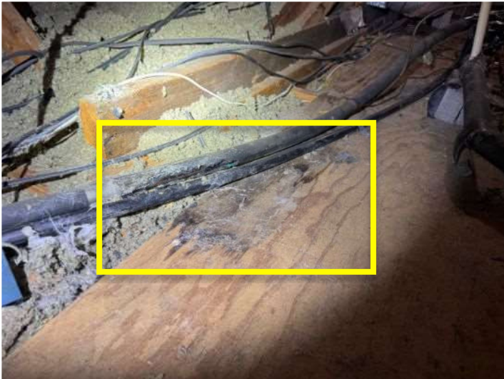
Condensation from refrigerant line in attic - Missing insulation - Water dripping
