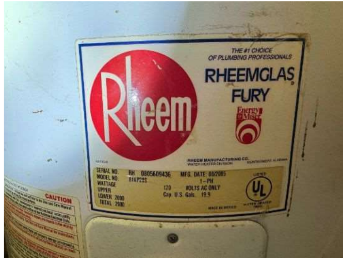
Data info - water heater 19.9 gallons.
