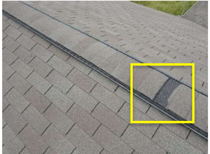
Damaged shingle
