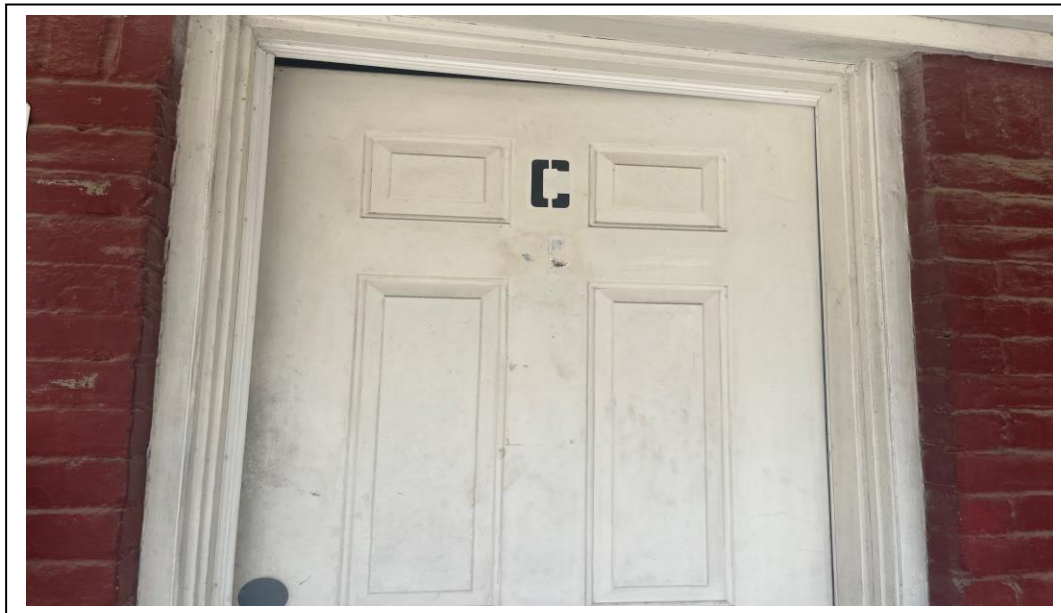
VIEW OF DOOR OF UNIT C
