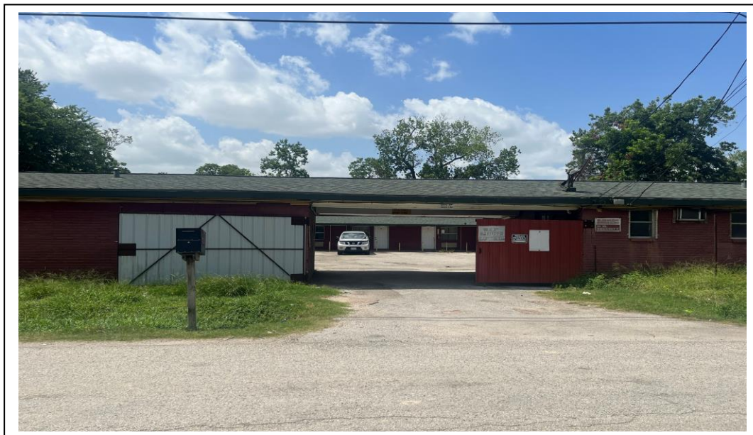
FRONT VIEW FROM RITZ DRIVE
