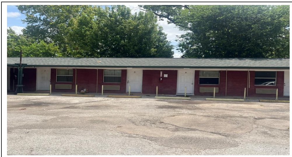
CONTINUED VIEW OF SOUTH SIDE OF BUILDING
