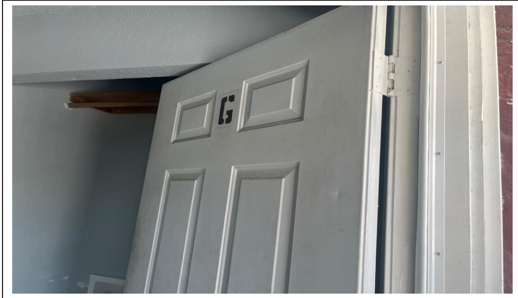
VIEW OF DOOR OF UNIT G
