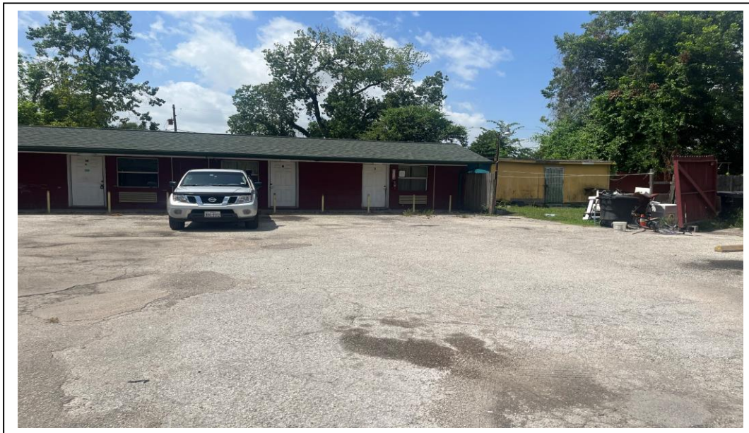
VIEW OF EXTERIOR SOUTH EXTERIOR WING OF SUBJECT
