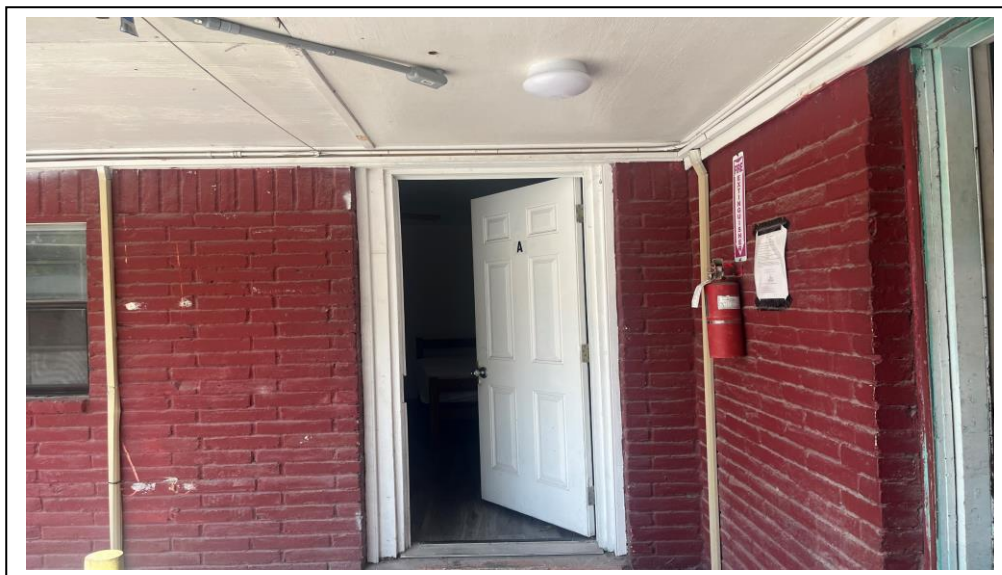
VIEW OF FRONT DOOR OF UNIT A
