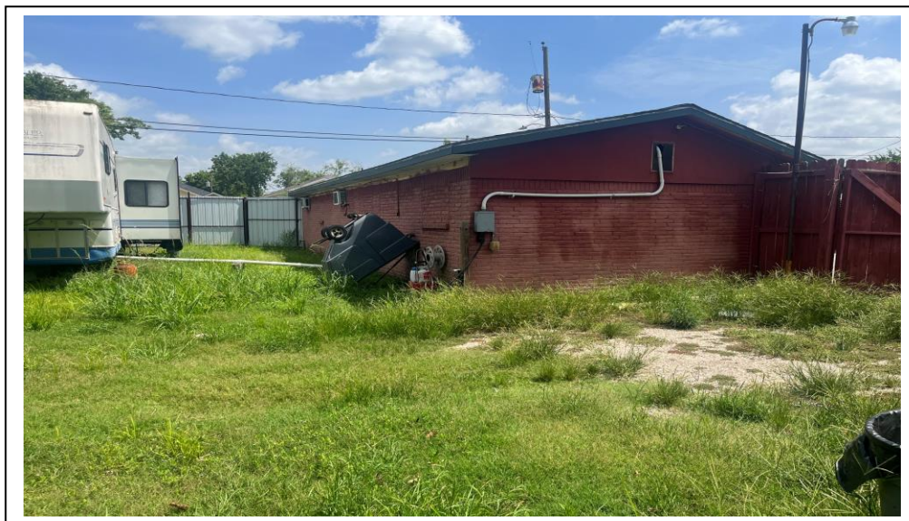
VIEW OF EXTERIOR WEST SIDE OF SUBJECT
