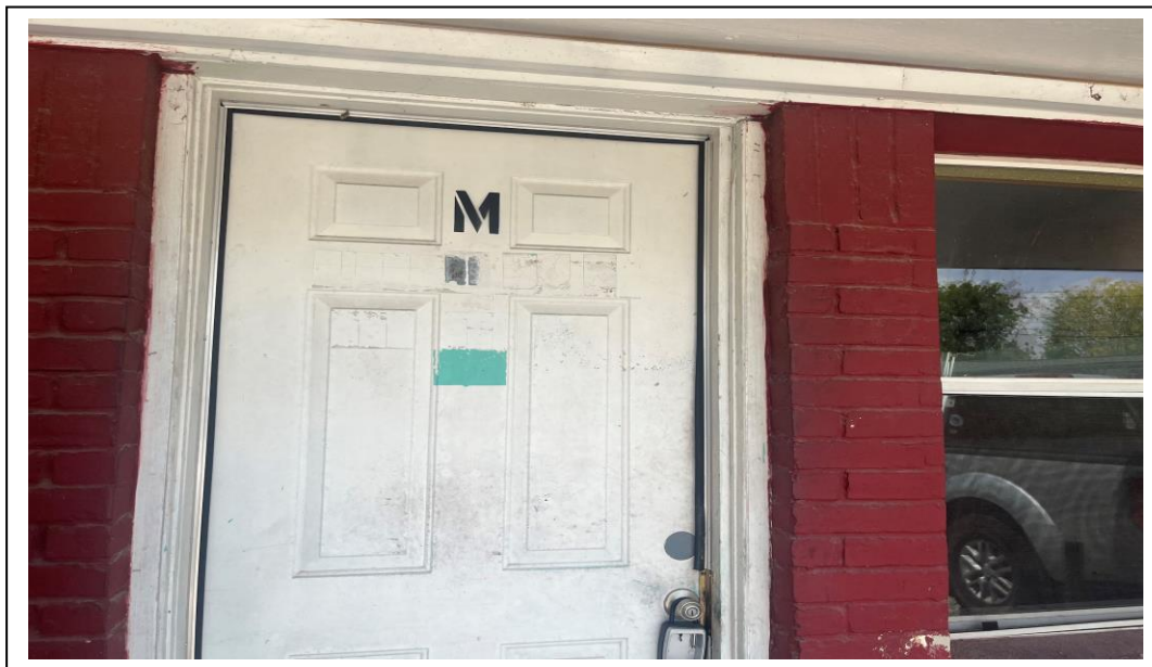
FRONT DOOR VIEW UNIT M
