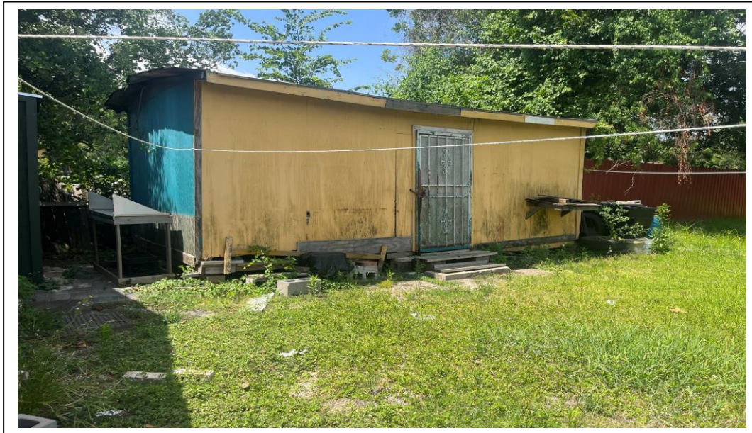
VIEW OF LARGE WORKSHOP/SHED AREA
