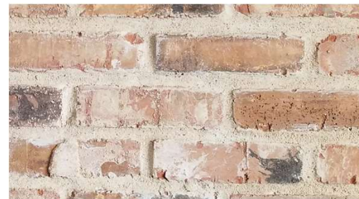
EXPOSED BRICK ACCENTS + FRONT PATIO FLOOR
