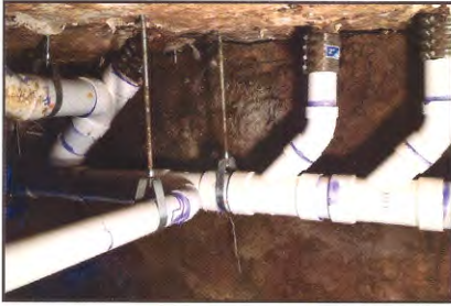
REMOVE & REPLACE CAST IRON WITH PVC
