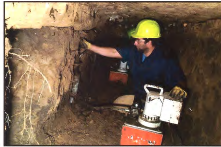
DRIVING PILES TO SUPPORT BEAMS
