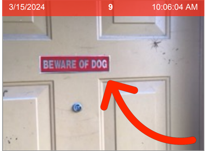
Front Door Exterior | Sticker on door
