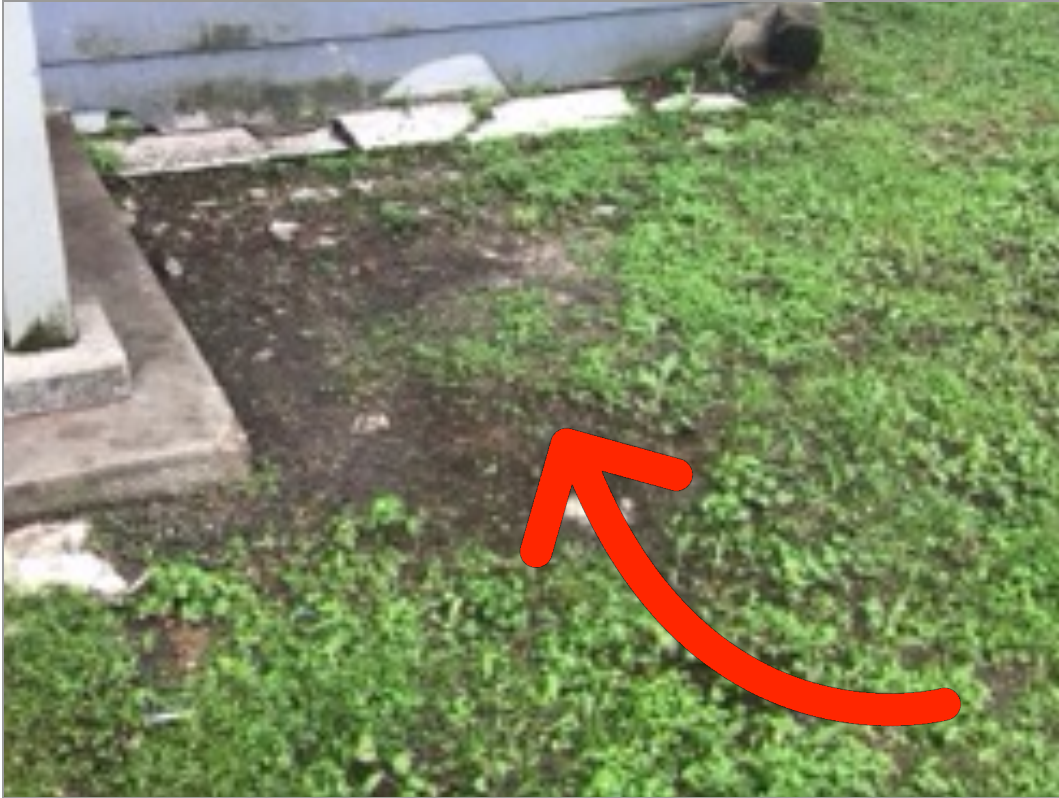
Front Exterior Yard Patches/dead spots in the grass
