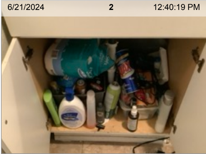
Cabinet Under Sink
