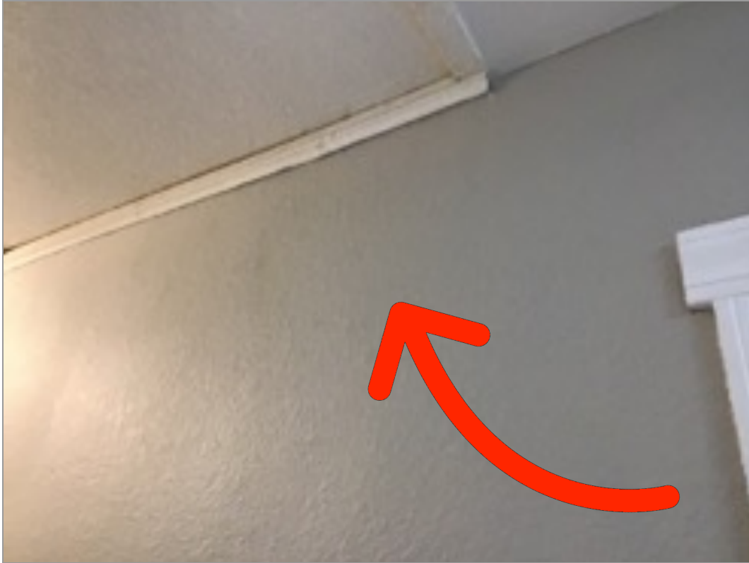
Hallway/Stairway Smoke Alarm Alarm in place
