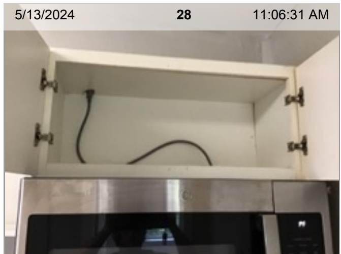
Upper Cabinets - Interior
