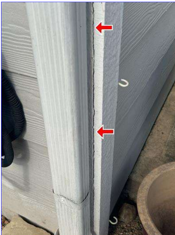
(2) Areas were observed, where the brick, stone, stucco, siding and/or trim needs to be sealed.
