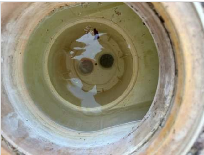
Skimmers were in good condition
