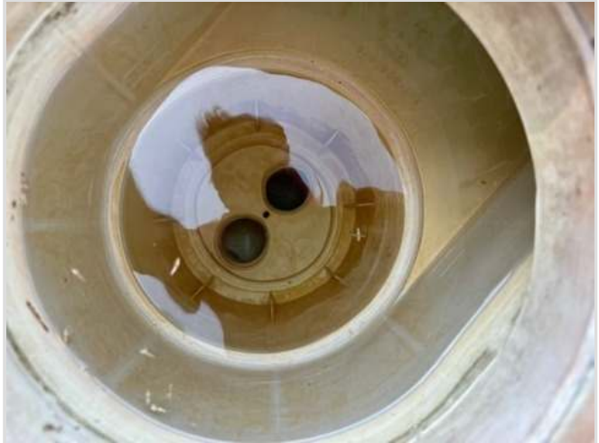
Skimmers were in good condition
