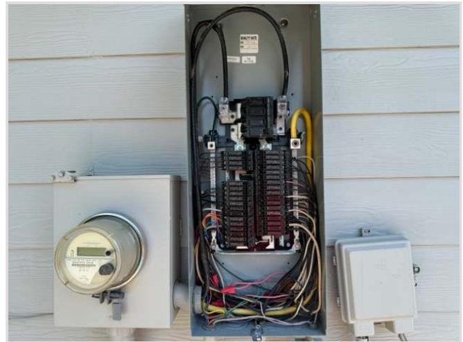
Cover removed for inspection
