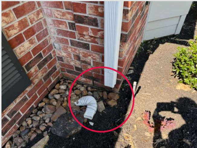
Bottom piece detached from downspout
