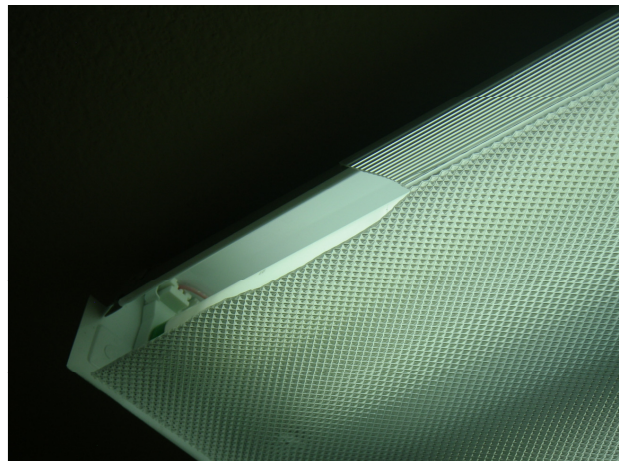
Picture of recessed light not secured to ceiling over master bathroom shower and picture of damaged lens cover on fluorescent light fixture in master closet.
