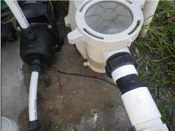
Picture of water leaking on concrete pad around pool/spa pump and motor. Picture of chlorinator leaking.
