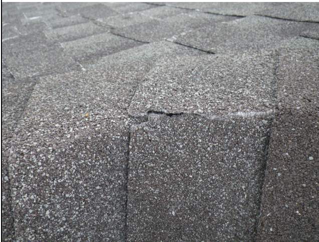
Sample pictures of cracked ridge shingles observed on roof.
