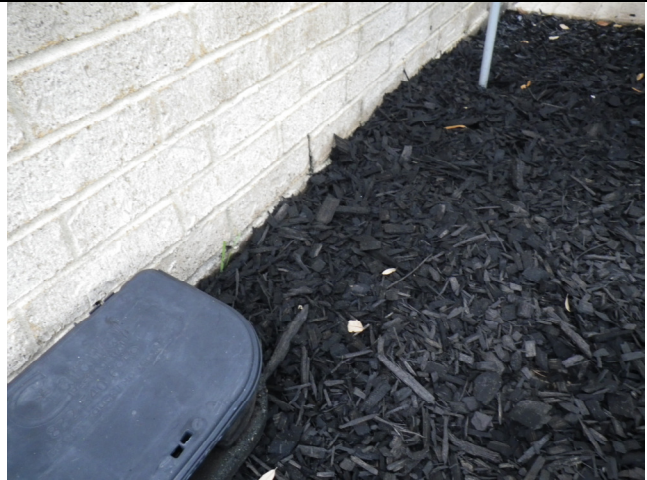
Sample pictures of high soil levels (built up bark mulch) in front flower beds.
