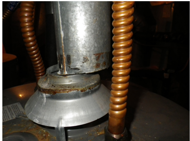
Picture of flue vent pipe at right side water heater not strapped in place where flue vent pipe terminates roof structure and picture of flue vent pipe not properly installed over draft diverter at left side water heater.
