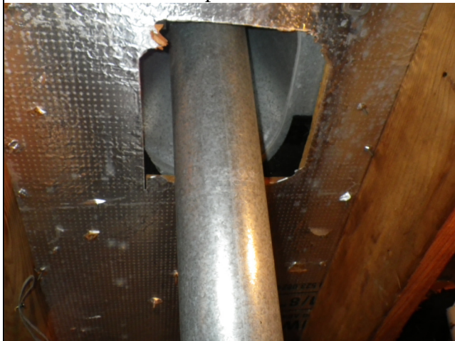
Picture of flue vent pipe at right side water heater not strapped in place where flue vent pipe terminates roof structure and picture of flue vent pipe not properly installed over draft diverter at left side water heater.
