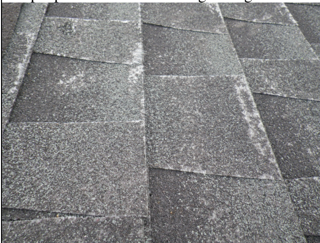
Sample pictures of shingles starting to delaminate.
