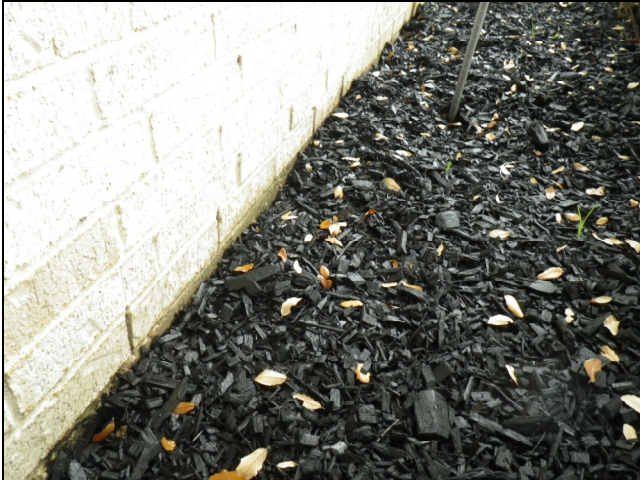
Sample pictures of high soil levels (built up bark mulch) in front flower beds.
