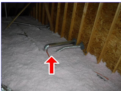
H. Item 1(Picture) Dryer duct to the outside
