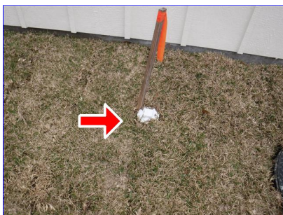
B. Item 1(Picture) Cleanout located on left side
