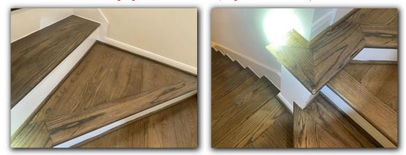
Warped / buckled wood floors were found in the Formal Living Room. A qualified tradesman should be consulted to determine the source of moisture and needed repairs.
