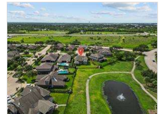
This aerial photo showcases a spacious, well-appointed suburban neighborhood with large single-family homes, manicured lawns, and an attractive community pond with a fountain feature. The area provides open green spaces and appears peaceful, ideal for those seeking a serene living environment.
