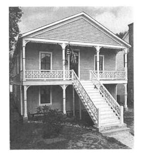
rehabilitation program. The house needed to be leveled, and an eightfoot hole in the roof and everything in between had to be repaired. All of the attic joists and rafters were rotted along with the sheathing and roofing shingles. The owners themselves hammered, sanded, painted and patiently cared for the fragile historic house.
