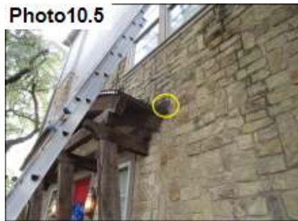
Kickout Flashing / Seal
