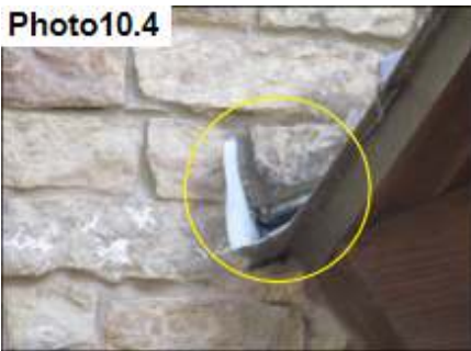
Kickout Flashing / Seal
