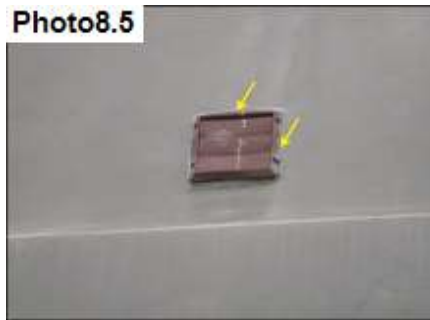
Penetration Sealants / Seal
