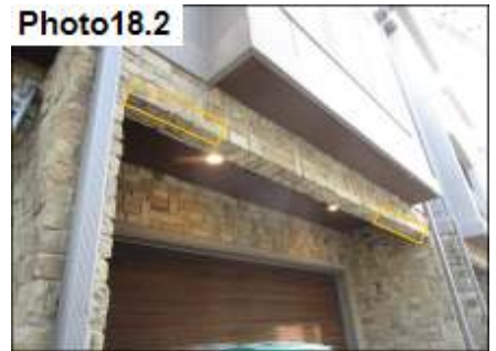
Deteriorated Mortar / Re-point
