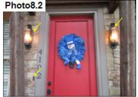
Penetration Sealants / Seal
