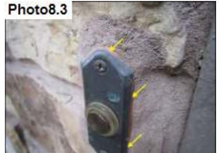
Penetration Sealants / Seal
