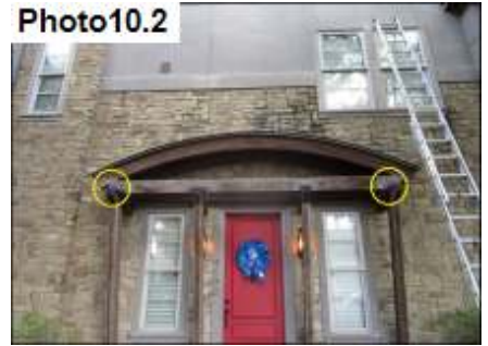
Kickout Flashing / Seal
