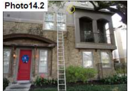
Kickout Flashing / Seal
