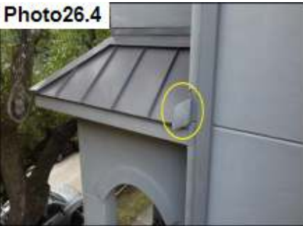
Kickout Flashing / Seal
