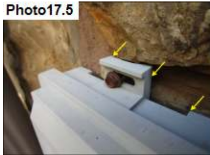
Penetration Sealants / Seal
