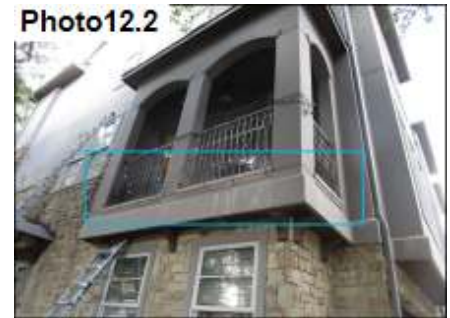
Balcony Flashing / Seal
