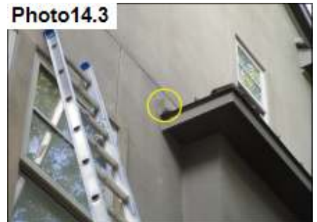
Kickout Flashing / Seal
