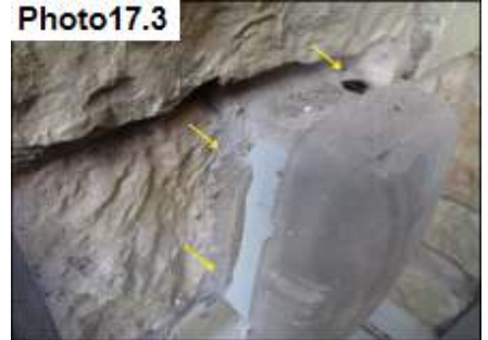
Penetration Sealants / Seal
