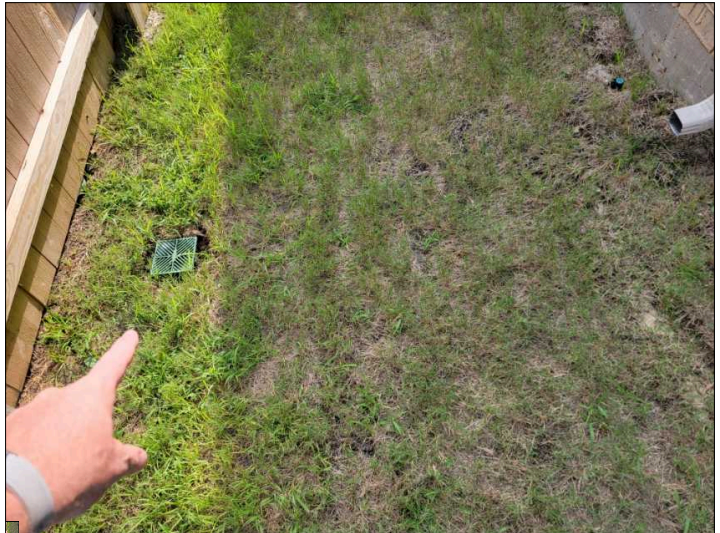
French drains are washed out around catch basin. Backfill as needed.
