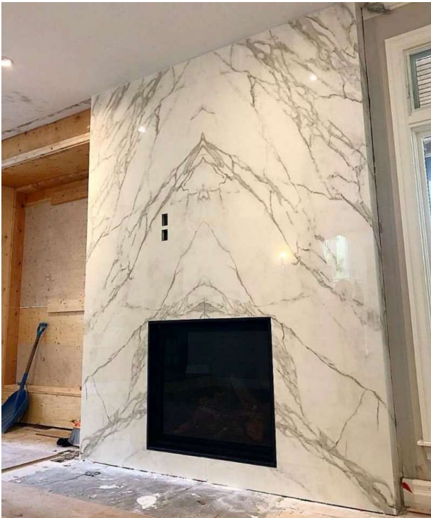
Booked Matched Porcelain Marble wrapped and matched on all sides above oversized fireplace in living room which compliments the exposed beams in kitchen
