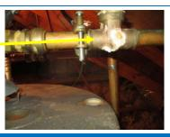
There was direct contact, or insufficient clearance between the water heater vent and the combustible roof decking. There should be at least 1" clearance between the Type "B" double wall vent pipe and the combustibles. The vent should be repositioned, or portions of the combustible material removed to allow the proper clearance.
