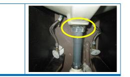
*Information:* Flexible drain lines are considered to be temporary repairs due to the propensitiy of the ridges to trap oils, hair, debris, etc. leading to blockage. There are corrugated drains which are smooth on the inside and are acceptable as drains.
