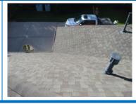
Information: Dish-type antenna was/were secured to the roof. Drilling holes through the roof damaged the roof cover and the gasket, caulk or sealant applied is not a guarantee against moisture penetration. Items mounted to the roof such as satellites, antennas, basketball backboards, etc., may allow water penetration. As these items move (wind, adjustments to position, use, etc.), screws and
