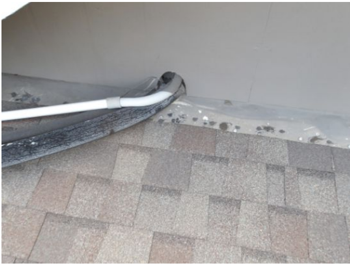
Enclose opening at roof level around a/c supply line into home
