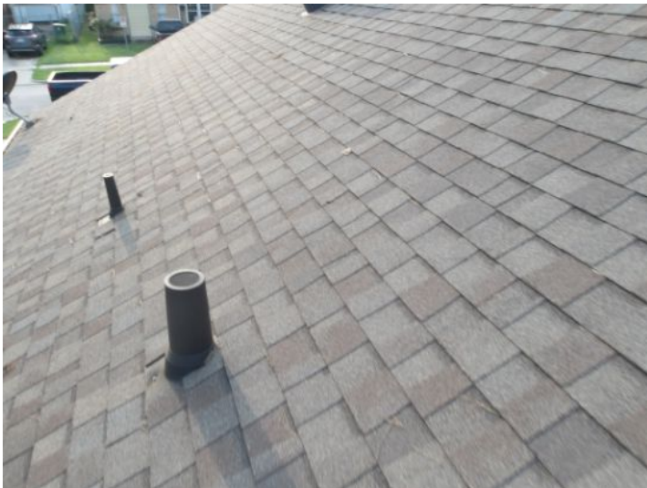
Roof covering was functioning as intended at the time of inspection
