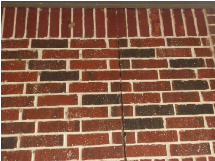
Reseal expansion joints
