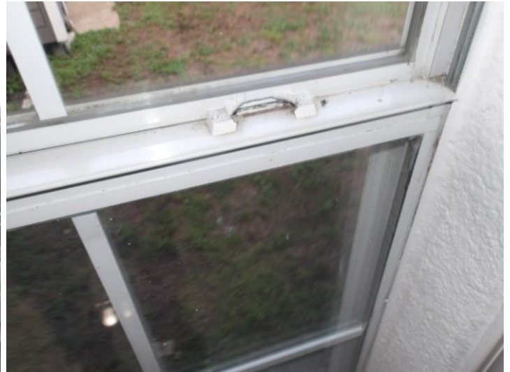
Broken locks on window in Laundry Room
