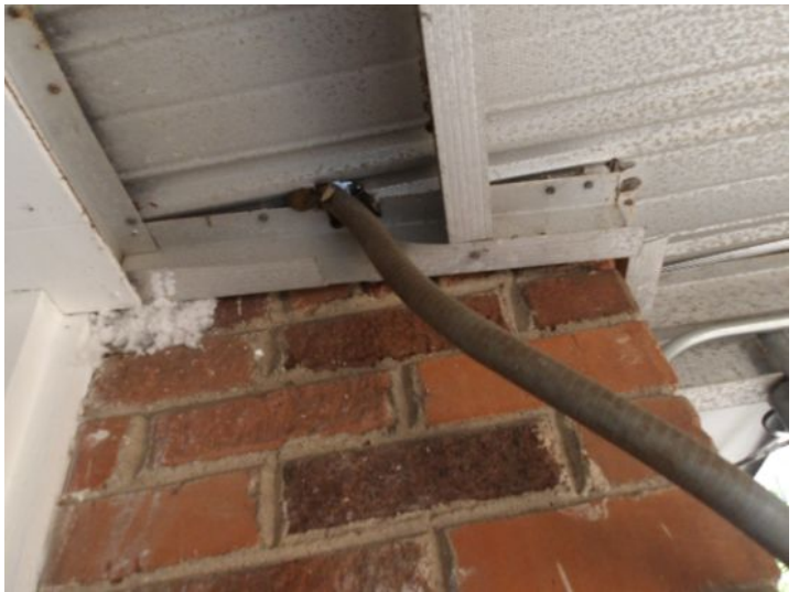
Enclose opening on carport at side of house
