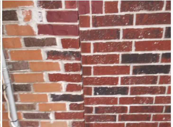
Reseal expansion joints
