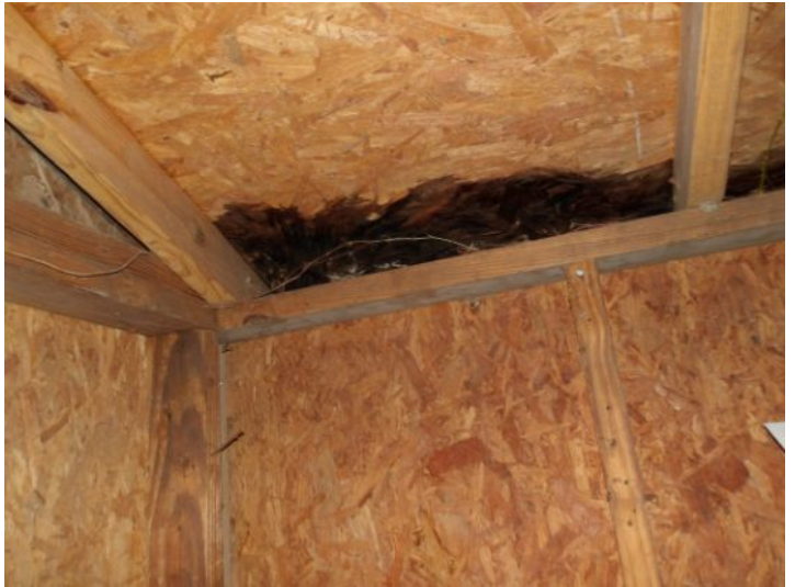
Rotted and damaged roof sheathing on Back shed
