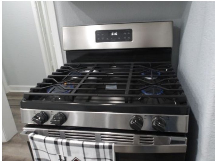
No anti-tilt device bracket present
