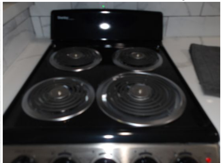
No anti-tilt device bracket present on oven in Back Building
