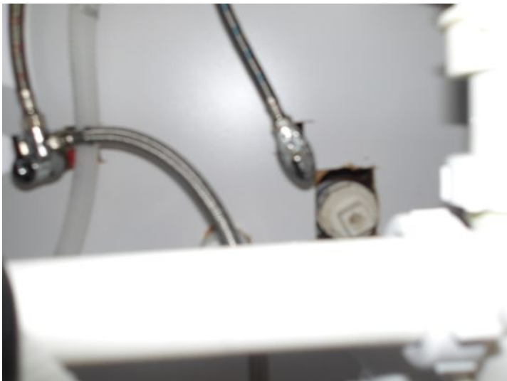
Enclose openings around kitchen sink supply and drain lines
