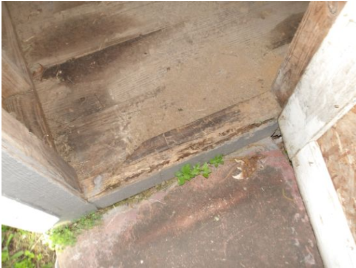
Rotted and damaged boards on Back shed
